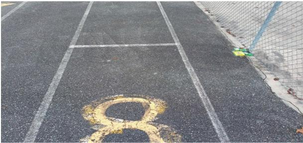
Two photos of current condition of the track. Cracks, weed and grass encroachment, general deterioration.
