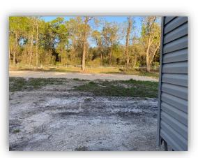
The finished floor of the home is below the required elevation of one foot above the adjacent road. The topography of the site drains to the northwest from the building site. There are no wetlands and flood plains on the property.
