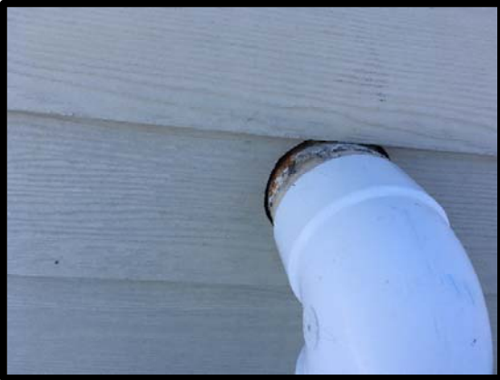
Picture 9: Typical penetration in Hardi plank
