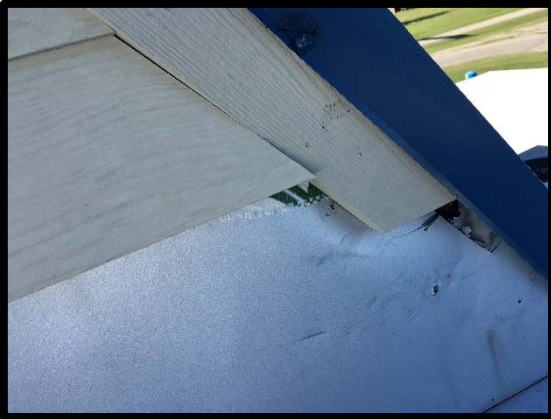
Picture 5: Limited Tyvek behind Hardi plank
