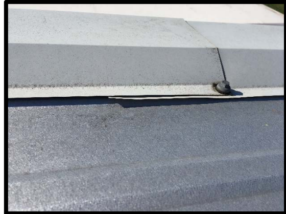
Picture 6: Overlapping of metal decking
