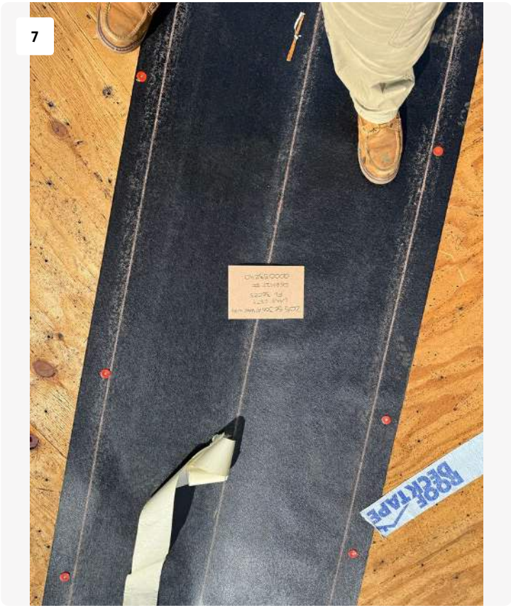
Project: Inspection Photos 205 Se Jonathan Date: Jul 1, 2025, 10:53 AM Creator: Logan Cotton
