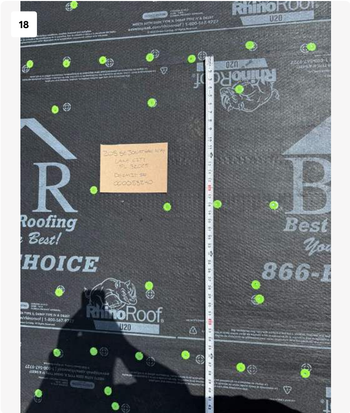
Project: Inspection Photos 205 Se Jonathan Date: Jul 1, 2025, 12:01 PM Creator: Logan Cotton
