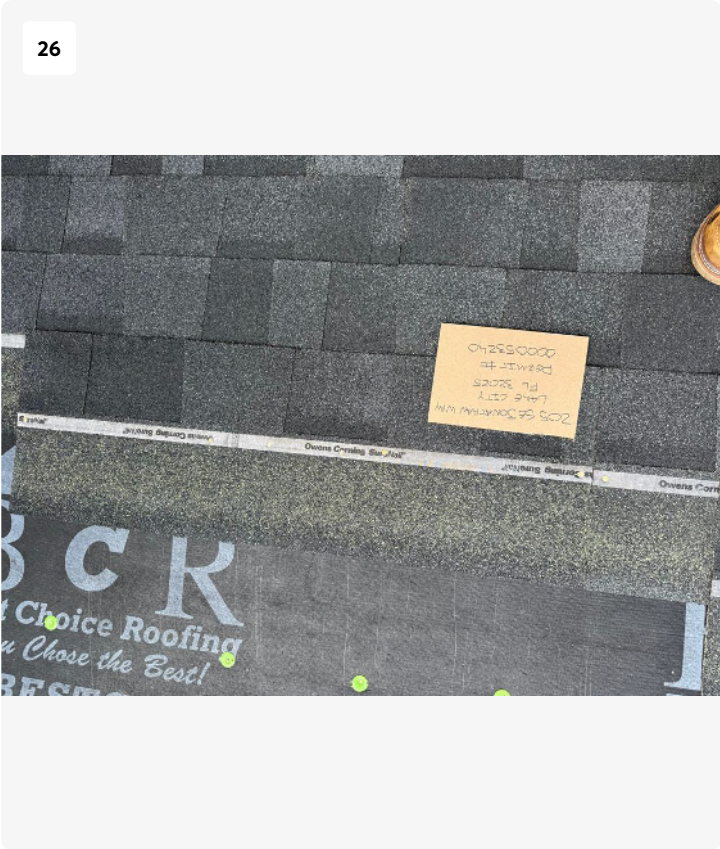
Project: Inspection Photos 205 Se Jonathan Date: Jul 1, 2025, 3:32 PM Creator: Logan Cotton
