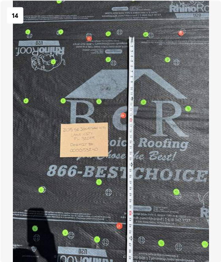
Project: Inspection Photos 205 Se Jonathan Date: Jul 1, 2025, 11:58 AM Creator: Logan Cotton
