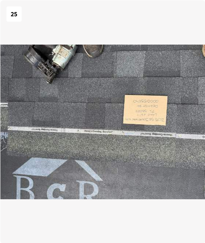
Project: Inspection Photos 205 Se Jonathan Date: Jul 1, 2025, 3:31 PM Creator: Logan Cotton
