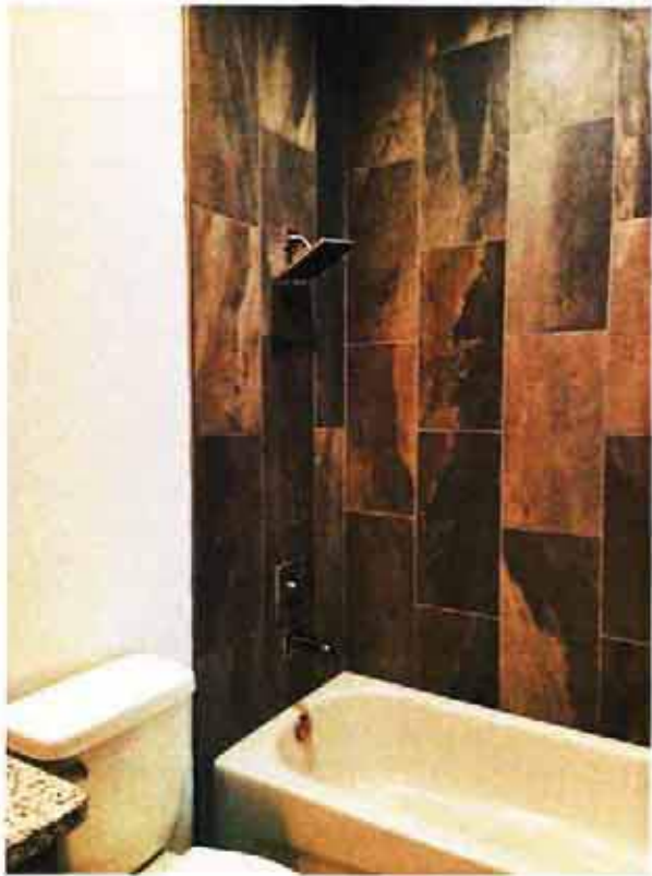
Tub/Shower Vertical Tile Detail
