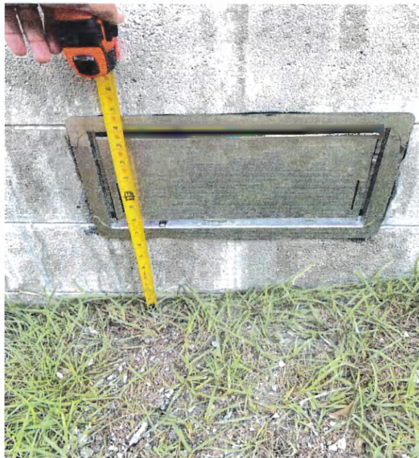
Foundation vent (front view)
