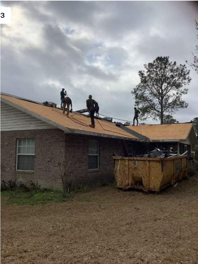
Project: 19156 US-441 Date: 2/18/2022, 9:47am Creator: Gary Solano
