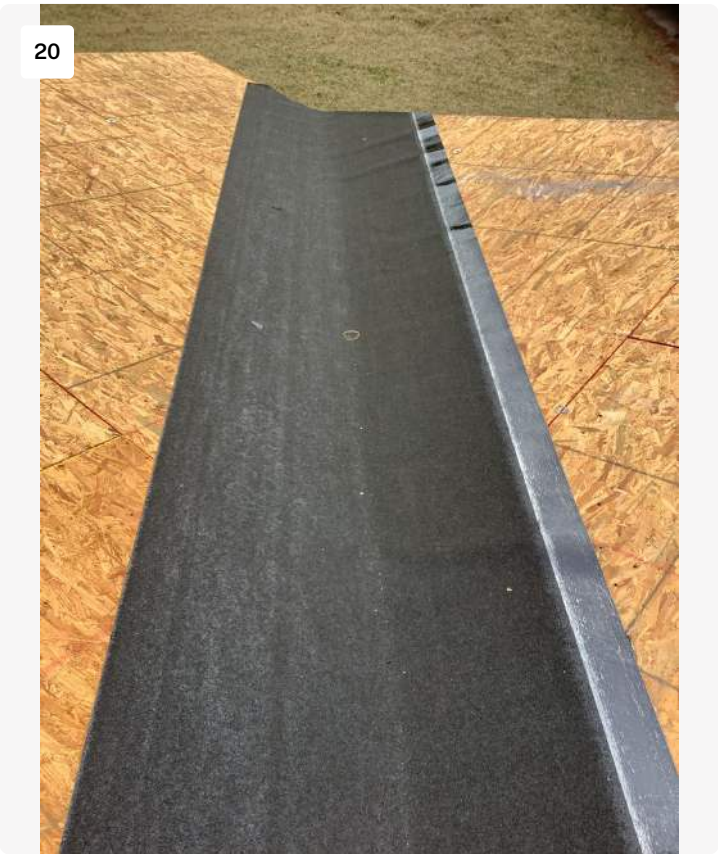
Project: 19156 US-441 Date: 2/18/2022, 10:31am Creator: Gary Solano
