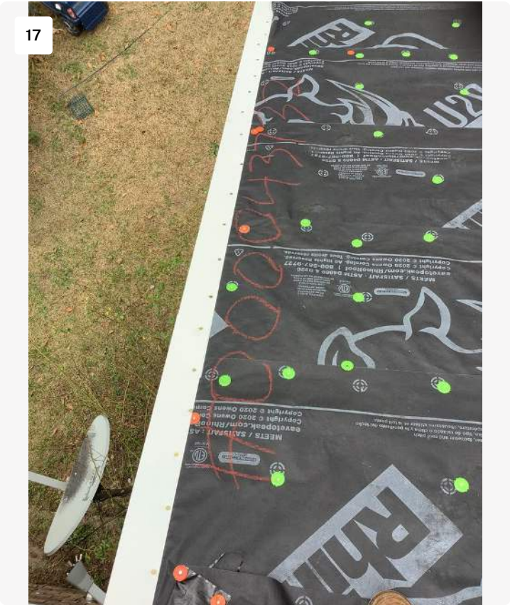
Project: 19156 US-441 Date: 2/18/2022, 10:29am Creator: Gary Solano
