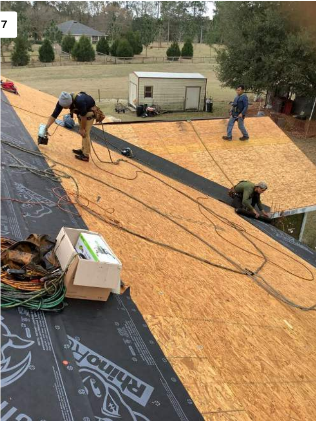
Project: 19156 US-441 Date: 2/18/2022, 9:49am Creator: Gary Solano
