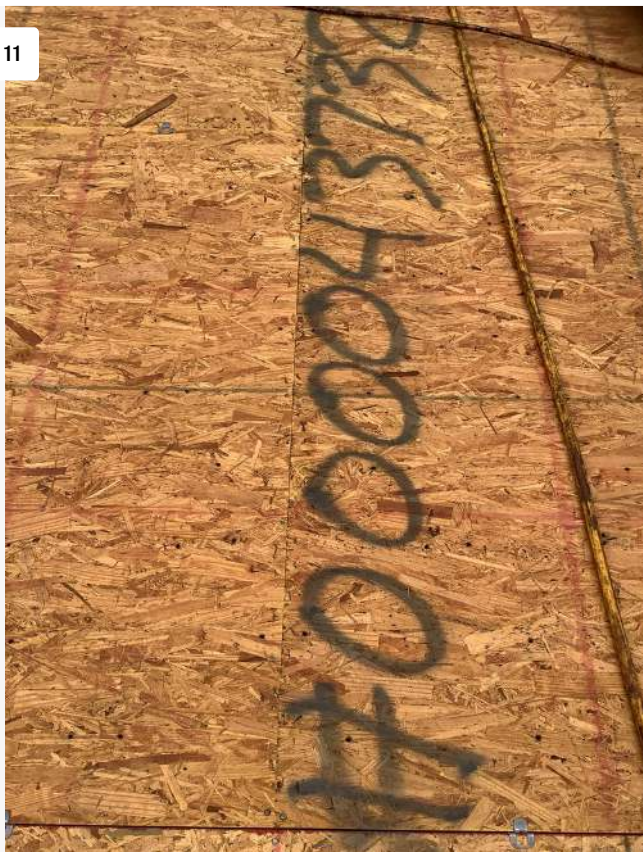
Project: 19156 US-441 Date: 2/18/2022, 10:24am Creator: Gary Solano
