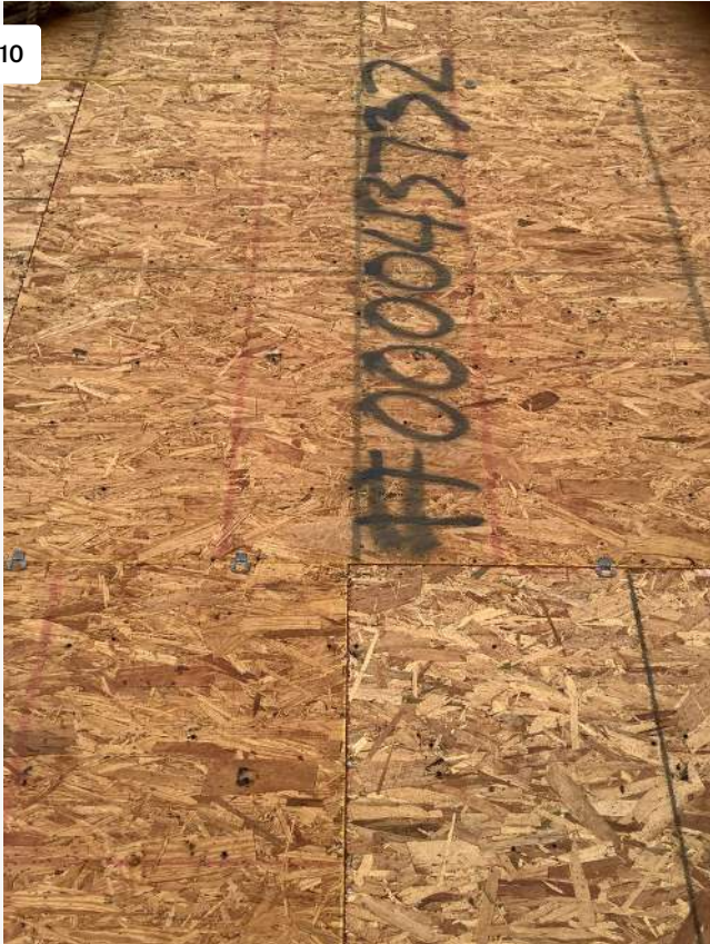
Project: 19156 US-441 Date: 2/18/2022, 10:12am Creator: Gary Solano
