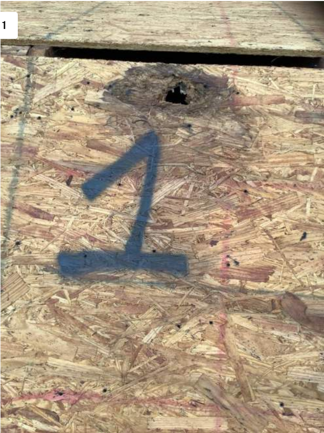
Project: 19156 US-441 Date: 2/18/2022, 9:20am Creator: Gary Solano
