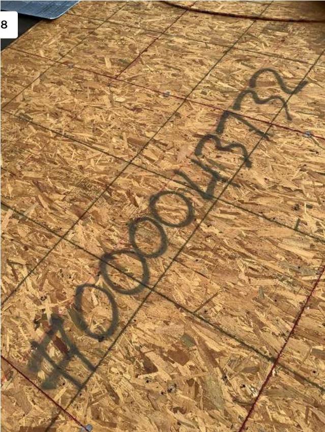
Project: 19156 US-441 Date: 2/18/2022, 10:06am Creator: Gary Solano
