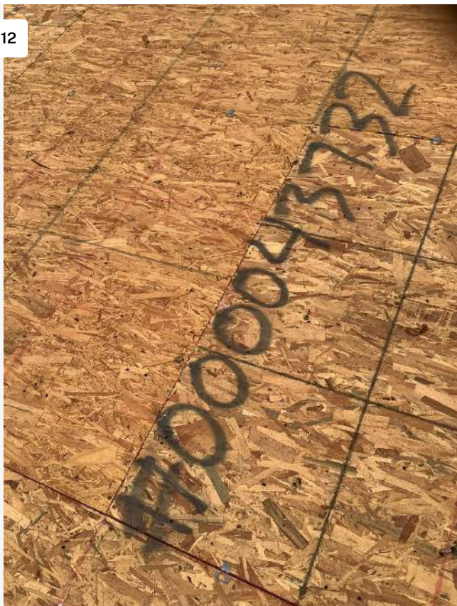
Project: 19156 US-441 Date: 2/18/2022, 10:25am Creator: Gary Solano
