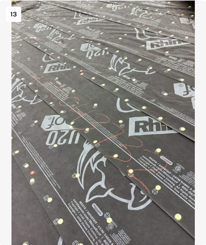
Project: 19156 US-441 Date: 2/18/2022, 10:26am Creator: Gary Solano
