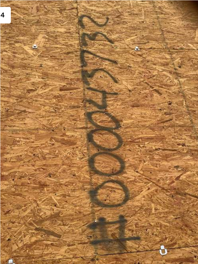
Project: 19156 US-441 Date: 2/18/2022, 9:48am Creator: Gary Solano
