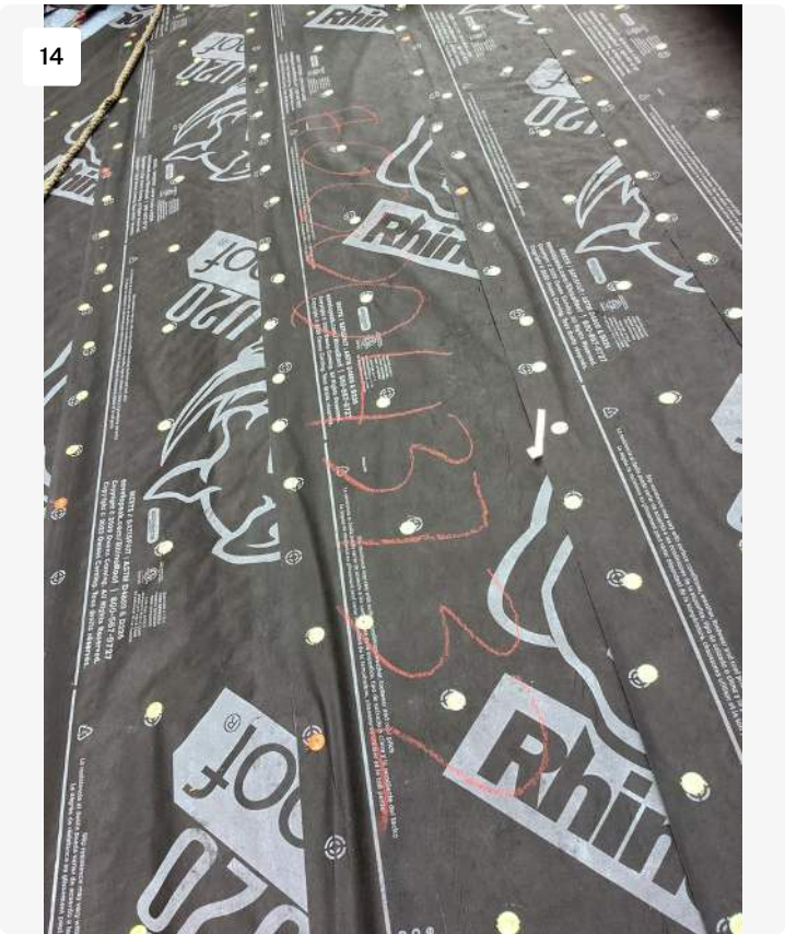
Project: 19156 US-441 Date: 2/18/2022, 10:28am Creator: Gary Solano
