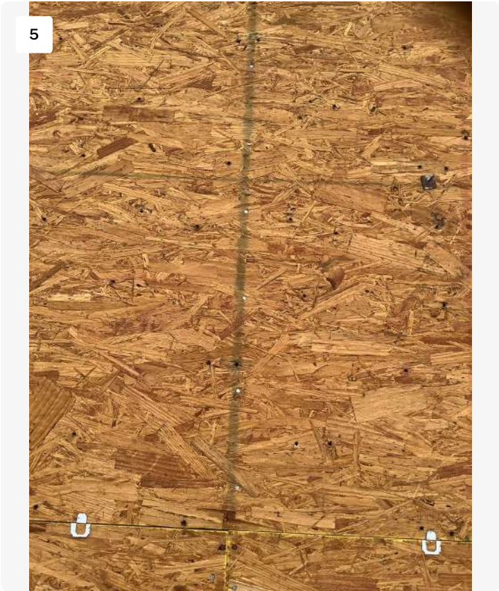
Project: 19156 US-441 Date: 2/18/2022, 9:48am Creator: Gary Solano
