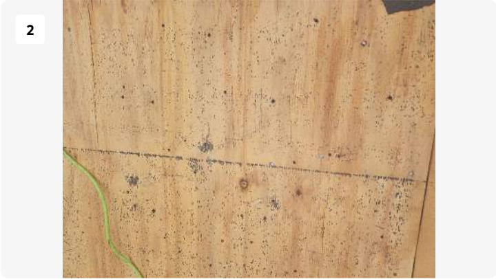
Project: 519 SW Lm Aaron Dr Date: 3/18/2024, 10:50am Creator: Jameson Fead Roofer
