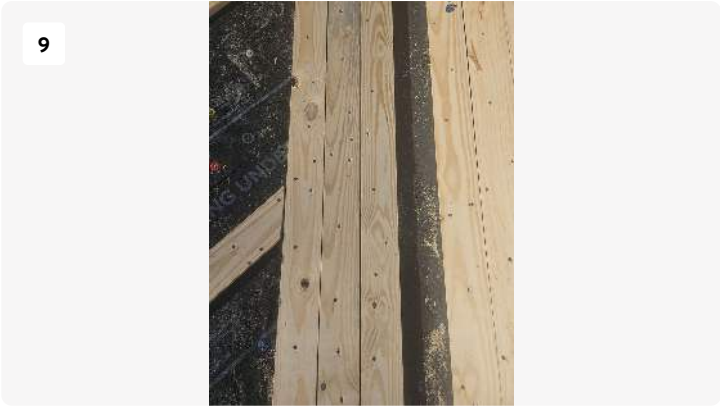
Project: 519 SW Lm Aaron Dr Date: 3/20/2024, 9:25am Creator: Jameson Fead Roofer
