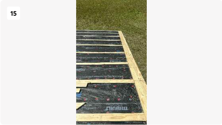
Project: 519 SW Lm Aaron Dr Date: 3/20/2024, 7:52pm Creator: Jameson Fead Roofer
