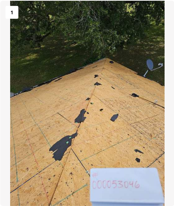
Project: 342 SW Legion Dr Lake City, FL 32024 Date: May 13, 2025, 10:53 AM
