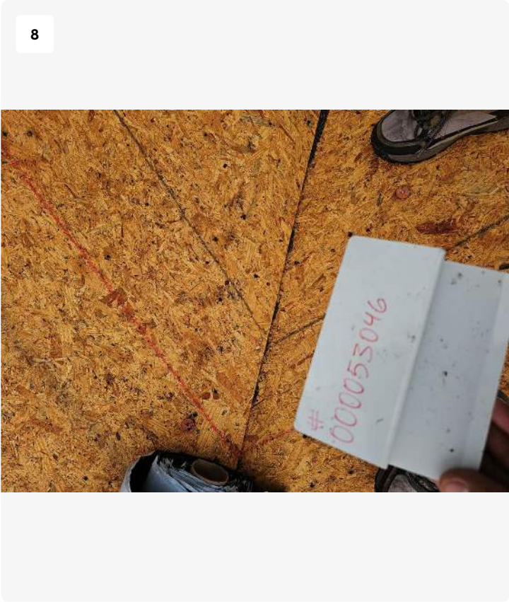
Project: 342 SW Legion Dr Lake City, FL 32024 Date: May 13, 2025, 12:17 PM
