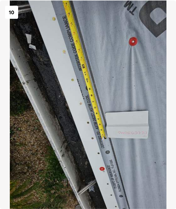
Project: 342 SW Legion Dr Lake City, FL 32024 Date: May 13, 2025, 4:14 PM
