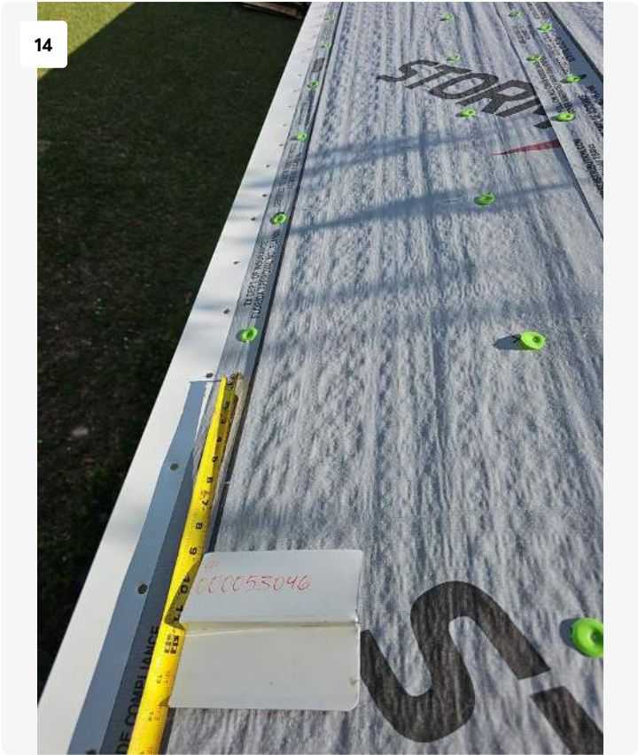
Project: 342 SW Legion Dr Lake City, FL 32024 Date: May 13, 2025, 5:21 PM
