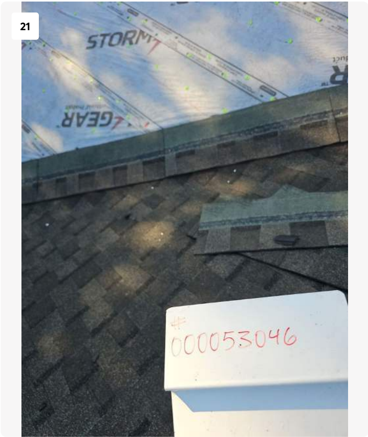
Project: 342 SW Legion Dr Lake City, FL 32024 Date: May 14, 2025, 8:22 AM
