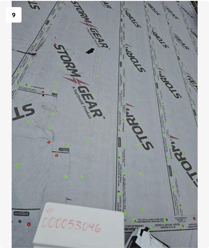
Project: 342 SW Legion Dr Lake City, FL 32024 Date: May 13, 2025, 4:09 PM
