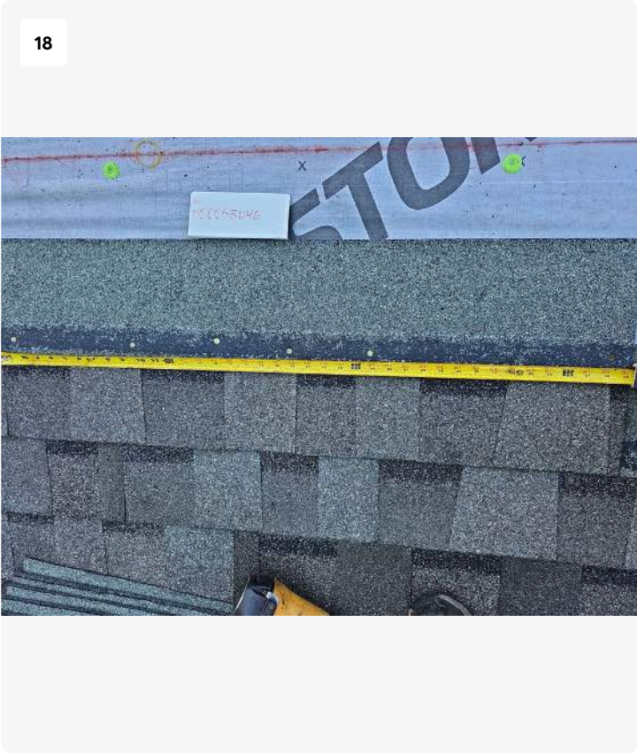
Project: 342 SW Legion Dr Lake City, FL 32024 Date: May 14, 2025, 8:21 AM
