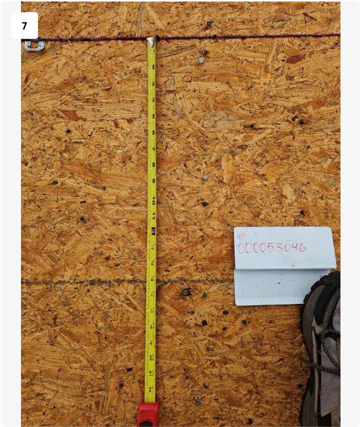
Project: 342 SW Legion Dr Lake City, FL 32024 Date: May 13, 2025, 12:15 PM
