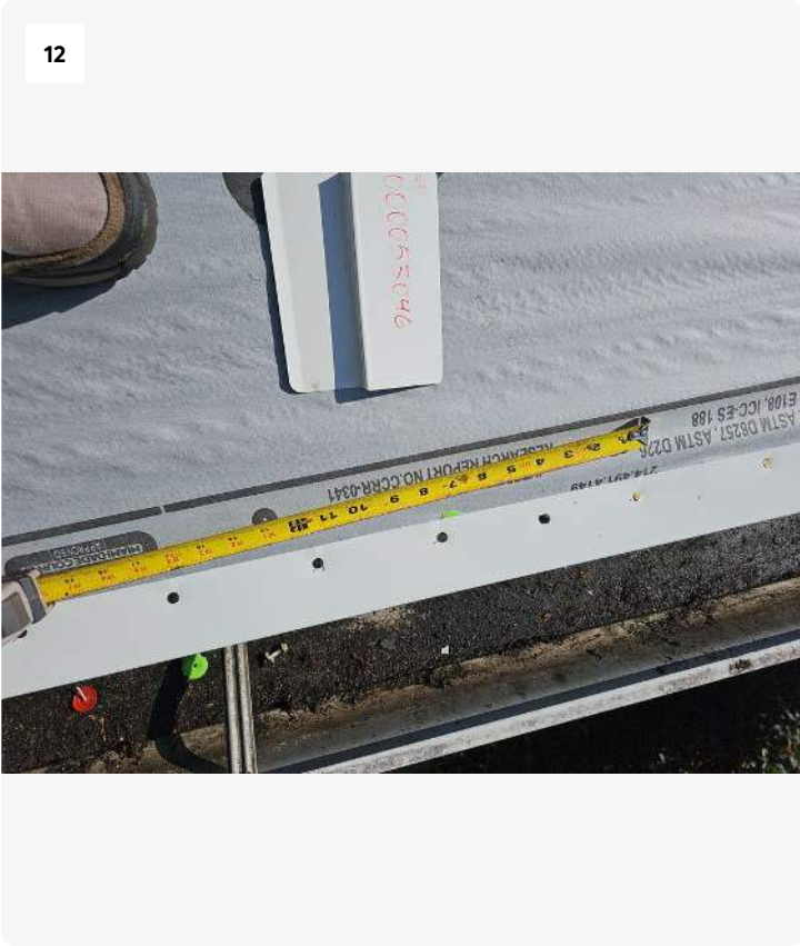
Project: 342 SW Legion Dr Lake City, FL 32024 Date: May 13, 2025, 5:20 PM
