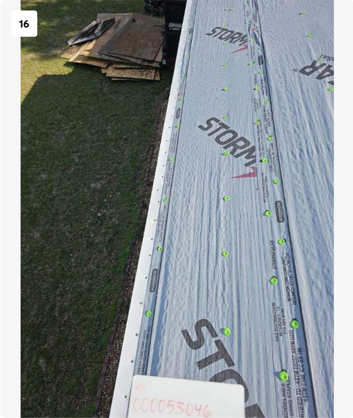
Project: 342 SW Legion Dr Lake City, FL 32024 Date: May 13, 2025, 5:22 PM
