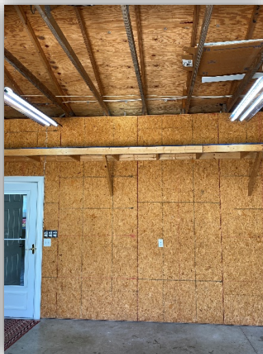
All-thread connectors exposed at interior wall separating garage from living space.
