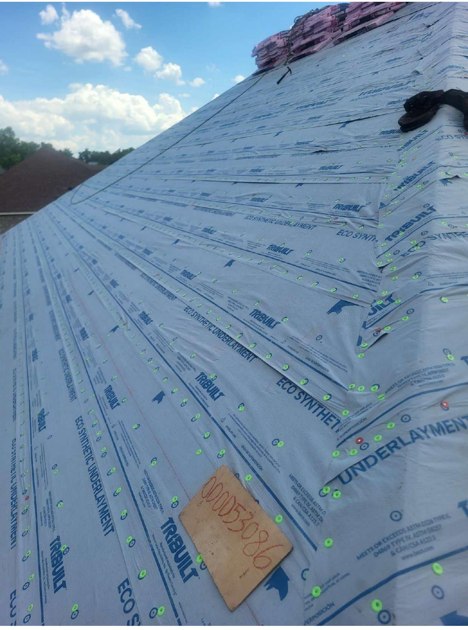
The image shows a steep roof under construction or renovation. Multiple layers of grey synthetic underlayment are laid down, with each layer featuring the 'TRIBUILT' logo in blue. A wooden clipboard with the handwritten number '000053086' is placed on one of the layers. The background features a bright blue sky with scattered white clouds and some green trees at the top of the hill.
