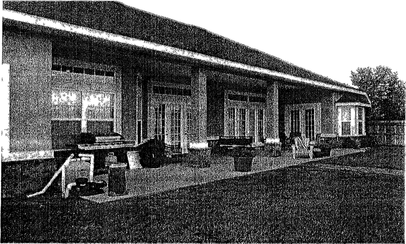
VIEW 3: BACK VIEW OF SUBJECT RESIDENCE (WEST SIDE)
