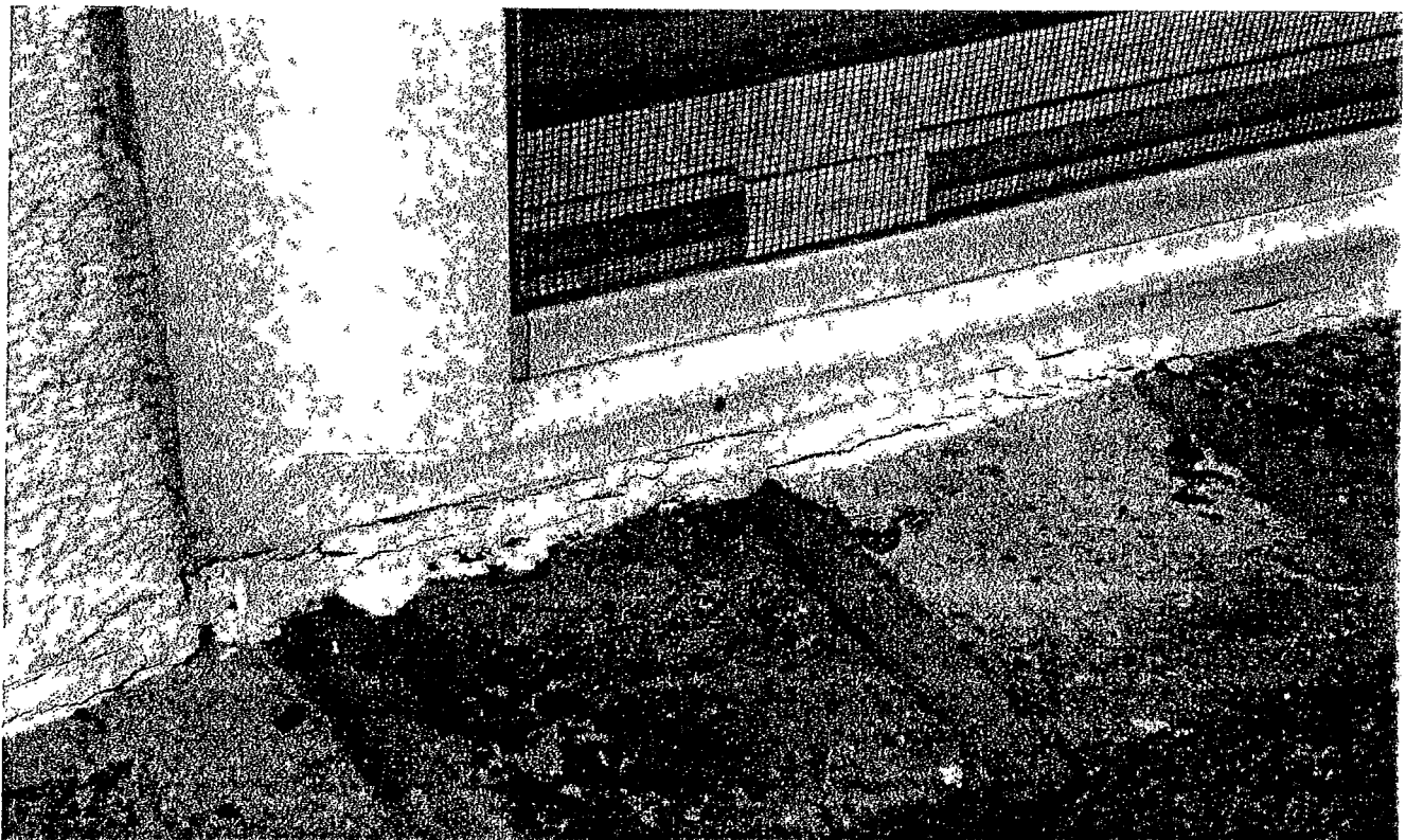
VIEW 26: WINDOW SEPARATION - BACK OF HOUSE - SOUTH BAY WINDOW, SOUTH END
