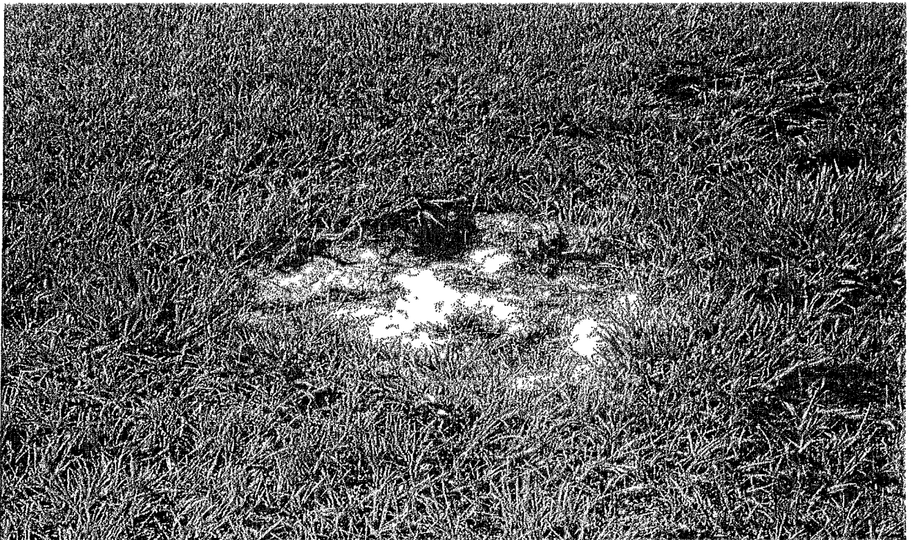
VIEW 28: VIEW OF DEPRESSION IN FRONT YARD - FILLED IN BY HOME OWNER
