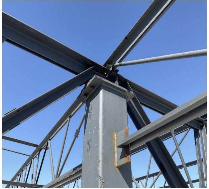
Tie plates not installed
