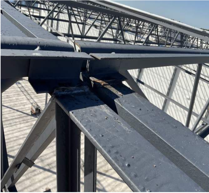
Typical joist welds
