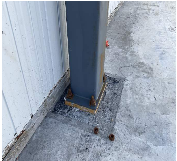
Base of column connections not tightened at time of inspection.
