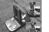
ATTACHING TO A RAFTER: Place FLASHLOC DUO over rafter location with sealant port on up-slope side and align upper edge of mount with horizontal chalk line. Secure mount with the two (2) provided rafter screws. BACKFILL ALL PILOT HOLES WITH SEALANT.
