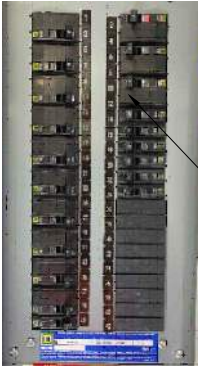
PROPOSED (1) 1P-15A BREAKERS IN POSITION 10 AND 12
