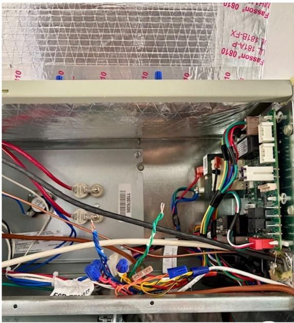
HVAC contractor is here installing the motorized damper to the make up air duct , the inspector asked to upload these photos to the portal also
