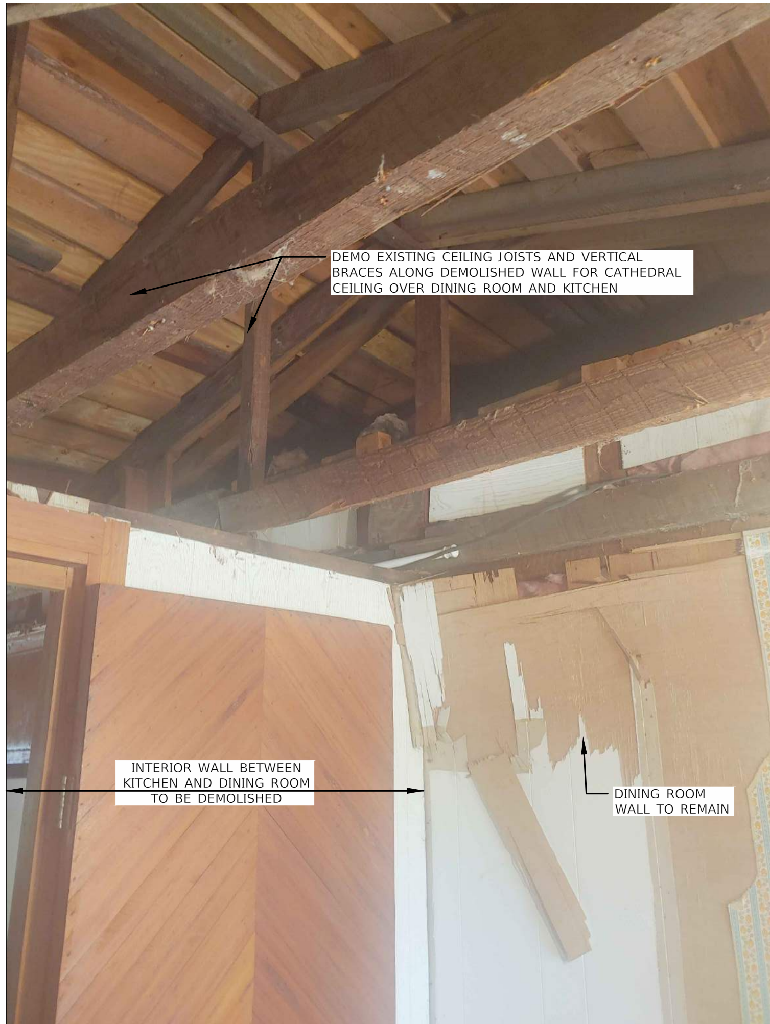
C DINING ROOM AREA REPAIR PHOTO DETAIL SCALE: N.T.S.
