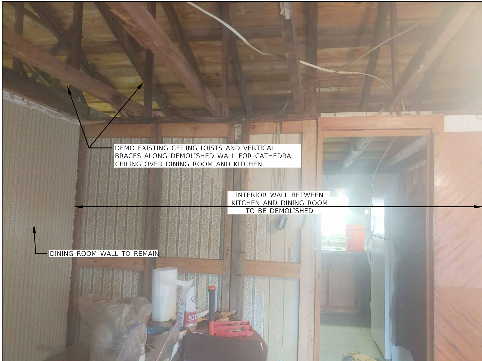
B DINING ROOM AREA REPAIR PHOTO DETAIL SCALE: N.T.S.
