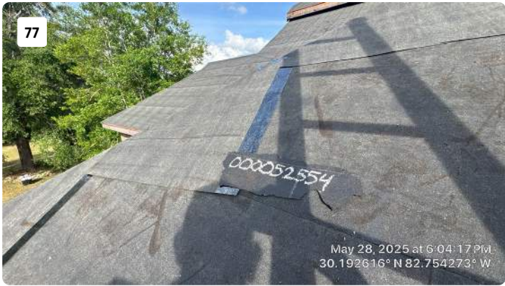
Project: 26706-088 Ordinario - Helene Date: May 28, 2025, 6:04 PM Creator: Stephen Kaywell
