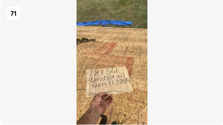
Project: 26706-088 Ordinario - Helene Date: May 28, 2025, 3:57 PM Creator: Stephen Kaywell
