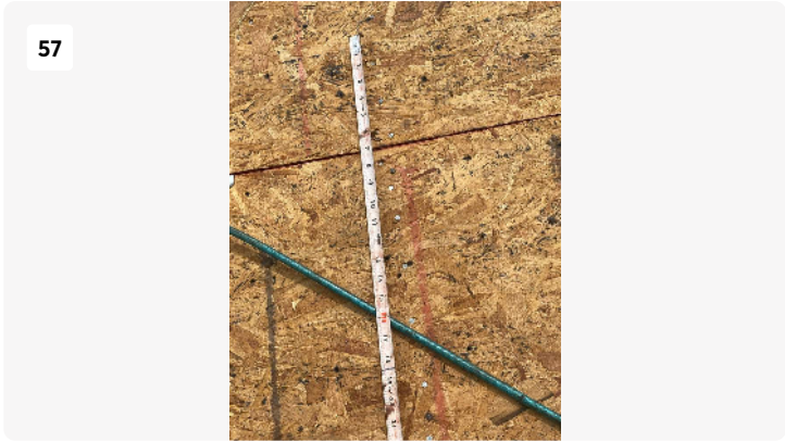
Project: 26706-088 Ordinario - Helene Date: May 28, 2025, 3:56 PM Creator: Stephen Kaywell
