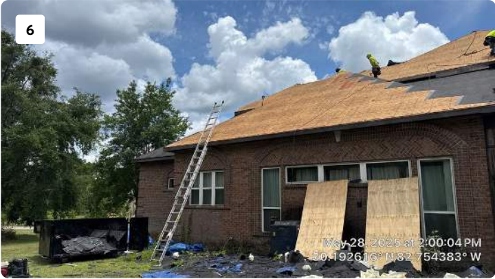
Project: 26706-088 Ordinario - Helene Date: May 28, 2025, 2:00 PM Creator: Stephen Kaywell
