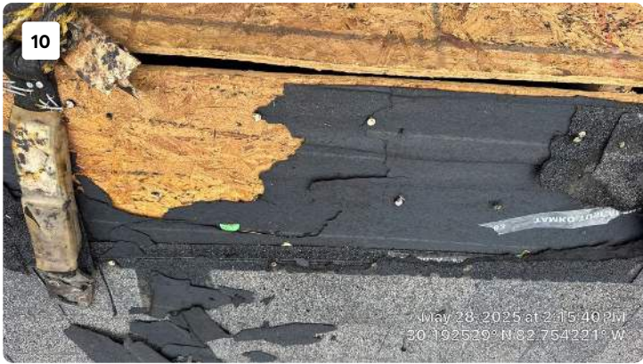
Project: 26706-088 Ordinario - Helene Date: May 28, 2025, 2:15 PM Creator: Stephen Kaywell
