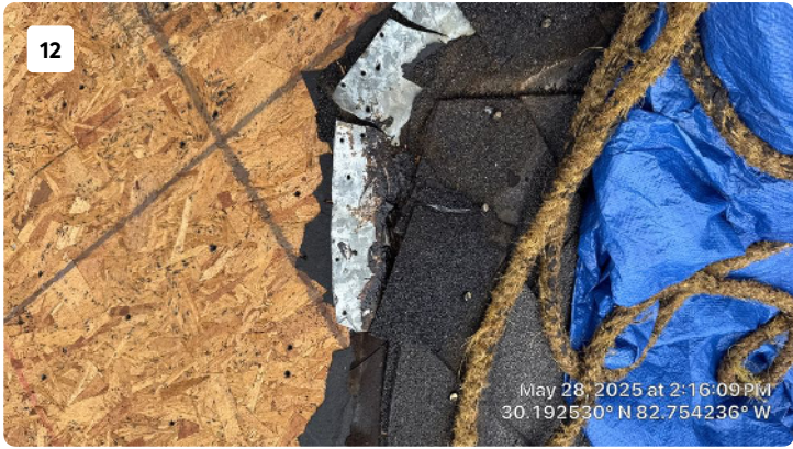
Project: 26706-088 Ordinario - Helene Date: May 28, 2025, 2:16 PM Creator: Stephen Kaywell
