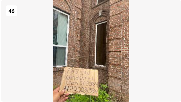
Project: 26706-088 Ordinario - Helene Date: May 28, 2025, 3:56 PM Creator: Stephen Kaywell
