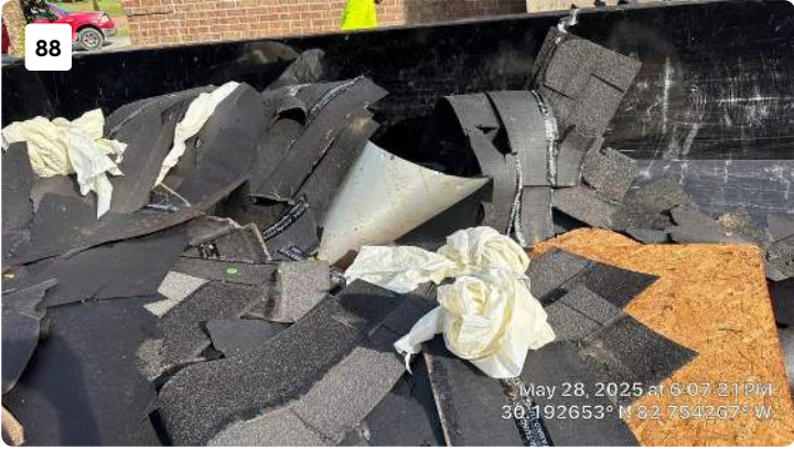
Project: 26706-088 Ordinario - Helene Date: May 28, 2025, 6:07 PM Creator: Stephen Kaywell
