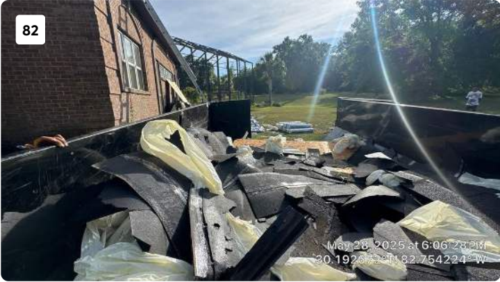
Project: 26706-088 Ordinario - Helene Date: May 28, 2025, 6:06 PM Creator: Stephen Kaywell
