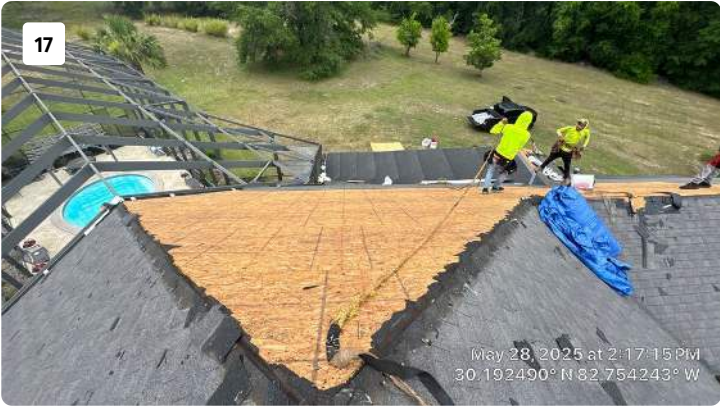
Project: 26706-088 Ordinario - Helene Date: May 28, 2025, 2:17 PM Creator: Stephen Kaywell
