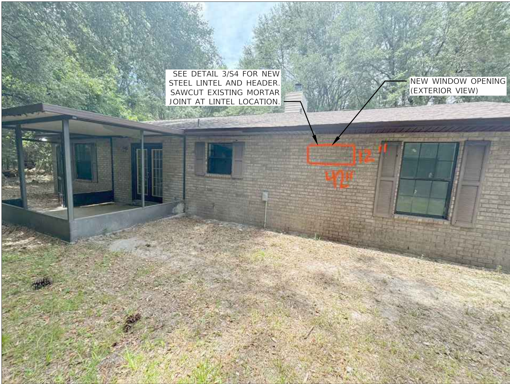
B BATHROOM REPAIR PHOTO DETAIL (EXTERIOR) SCALE: N.T.S.
