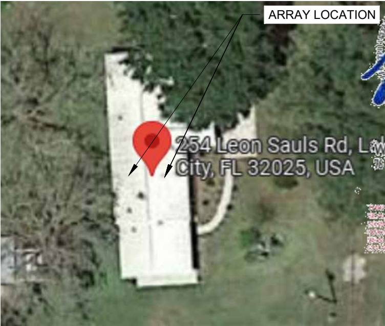
1 | HOUSE PHOTO PV-0 | SCALE: NTS
