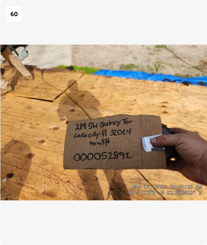
Project: 219 SW Quincy Terrace Date: May 16, 2025, 10:06 AM Creator: Joseph Knight
