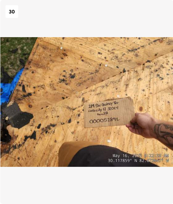
Project: 219 SW Quincy Terrace Date: May 16, 2025, 9:22 AM Creator: Joseph Knight
