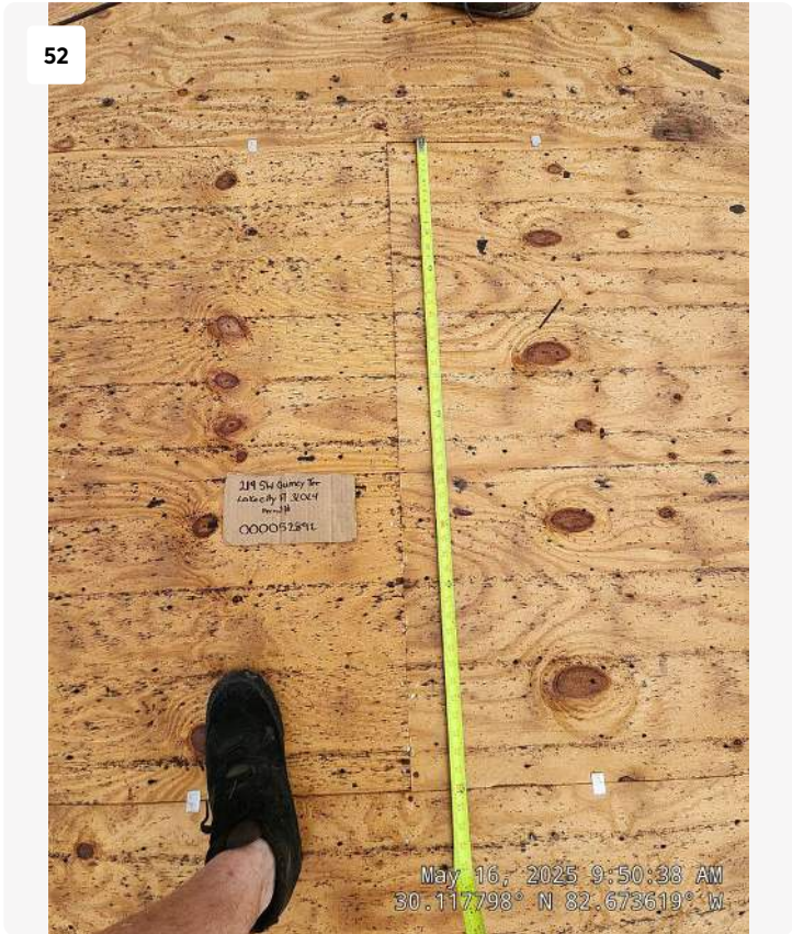
Project: 219 SW Quincy Terrace Date: May 16, 2025, 9:50 AM Creator: Joseph Knight
