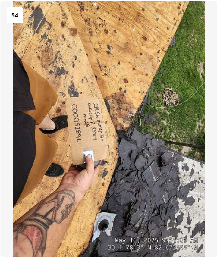
Project: 219 SW Quincy Terrace Date: May 16, 2025, 9:51 AM Creator: Joseph Knight
