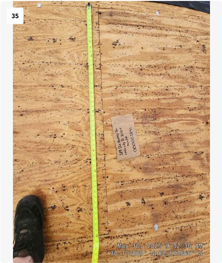
Project: 219 SW Quincy Terrace Date: May 16, 2025, 9:32 AM Creator: Joseph Knight
