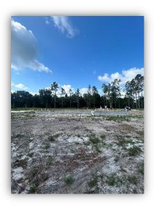
The topography of the site drains to the north. The finished floor elevation of the home shall be 12" above the adjacent ground for the entire perimeter of the foundation, except driveways and sidewalks. The finished floor of the home will be below required elevation of one foot above the adjacent road.
