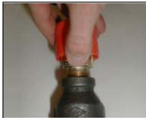
Figure 3: Sprinkler cap being removed from and upright sprinkler.
