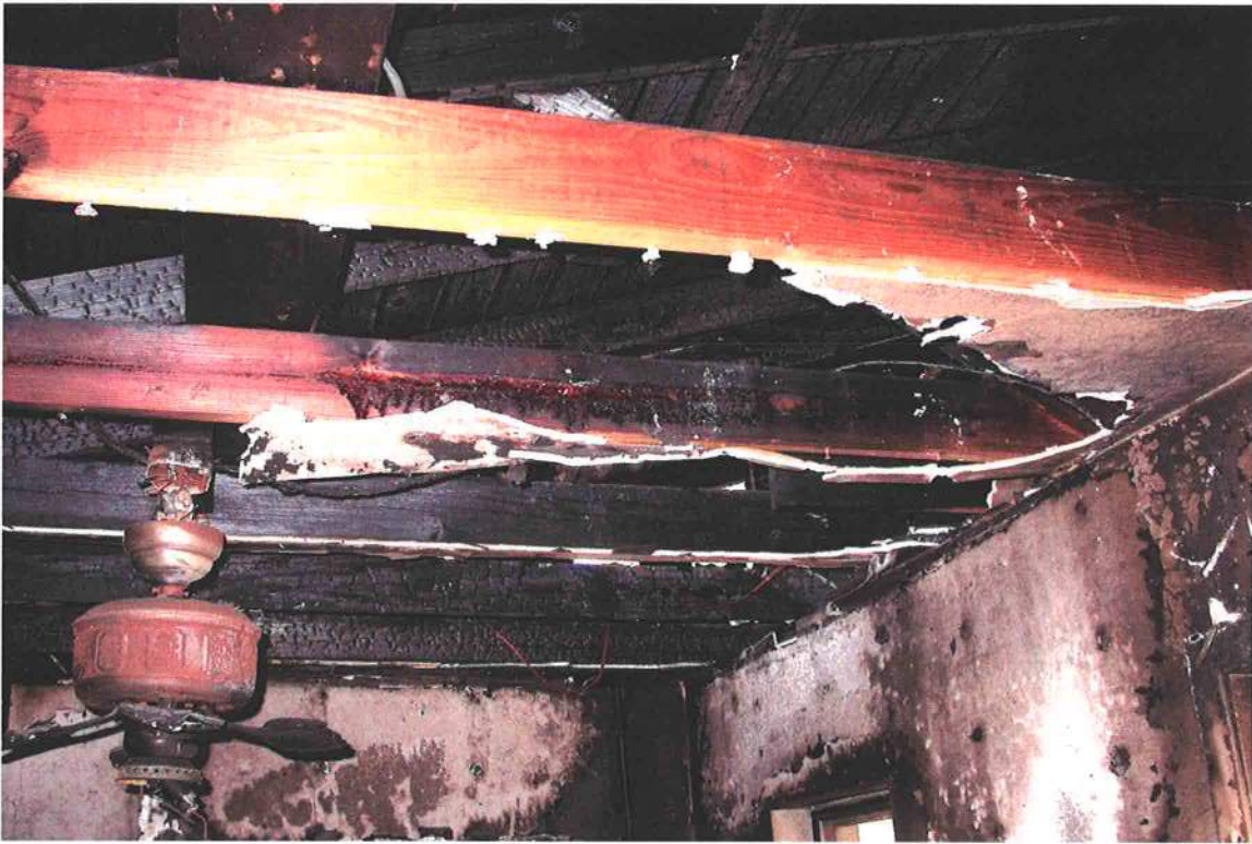
Photograph 3. View of damage to roof and ceiling framing over the kitchen.
