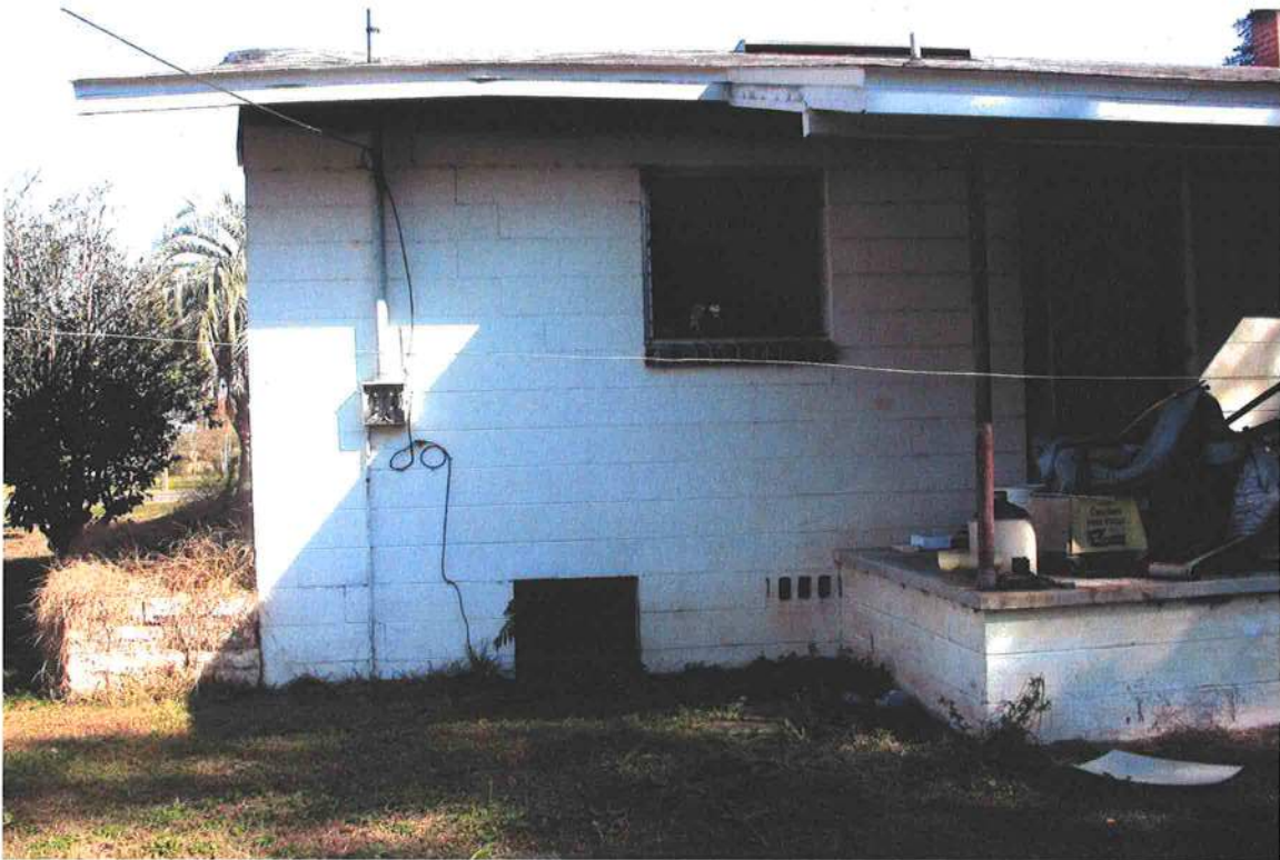
Photograph 2. View of damaged exterior wall near west corner of house. The top eleven courses should be removed and rebuilt from the corner to the southeast side of the window.
