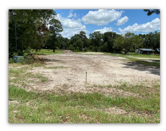
The minimum finished floor elevation for a structure constructed on the referenced site is 104.4. The elevation of the road adjacent to the site is 106.00 + /-. The design maximum stage elevation of the top of the adjacent basin per plan is 103.4. The existing ground elevation at building site is 103.0. The finished floor of the home will be at or below the nearest adjacent street.
