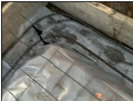
CORNER REINF'G ON CHAIRS W/ WIRE MESH AND PLASTIC VAPOR BARRIER
