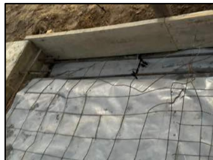
EDGE FTG INTERFACE W/ EXISTING SLAB
