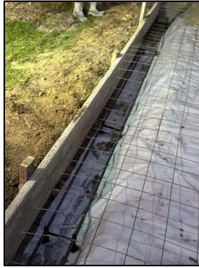
EDGE FTG W/ REBAR ON CHAIRS AND EDGE FORMING
