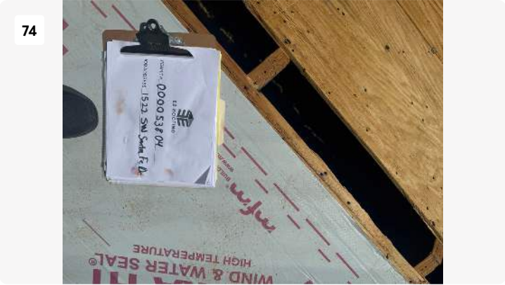
Project: Bruce & Natlie Park - SF GC Work Date: Sep 4, 2025, 12:18 PM Creator: kaleb carson
