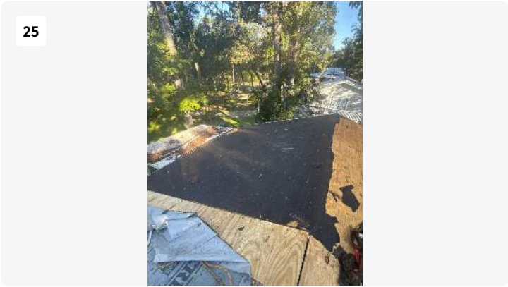
Project: Bruce & Natlie Park - SF GC Work Date: Sep 4, 2025, 9:04 AM Creator: kaleb carson
