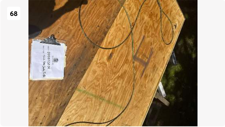
Project: Bruce & Natlie Park - SF GC Work Date: Sep 4, 2025, 12:01 PM Creator: kaleb carson
