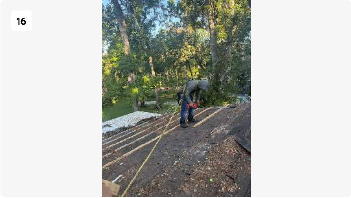
Project: Bruce & Natlie Park - SF GC Work Date: Sep 4, 2025, 8:35 AM Creator: kaleb carson
