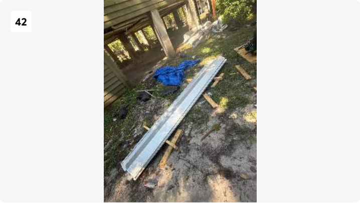
Project: Bruce & Natlie Park - SF GC Work Date: Sep 4, 2025, 11:14 AM Creator: kaleb carson
