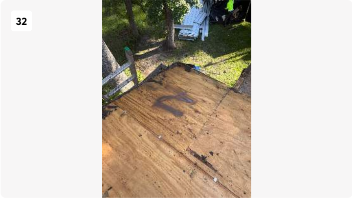
Project: Bruce & Natlie Park - SF GC Work Date: Sep 4, 2025, 9:16 AM Creator: kaleb carson
