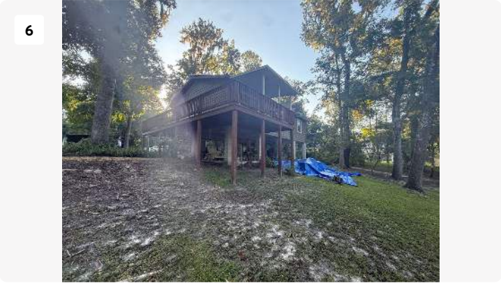
Project: Bruce & Natlie Park - SF GC Work Date: Sep 4, 2025, 8:20 AM Creator: kaleb carson
