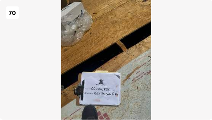
Project: Bruce & Natlie Park - SF GC Work Date: Sep 4, 2025, 12:17 PM Creator: kaleb carson
