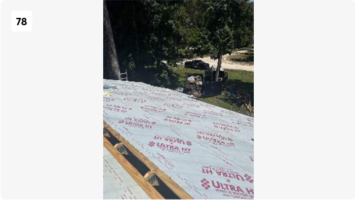
Project: Bruce & Natlie Park - SF GC Work Date: Sep 4, 2025, 1:32 PM Creator: kaleb carson
