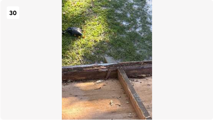
Project: Bruce & Natlie Park - SF GC Work Date: Sep 4, 2025, 9:13 AM Creator: kaleb carson
