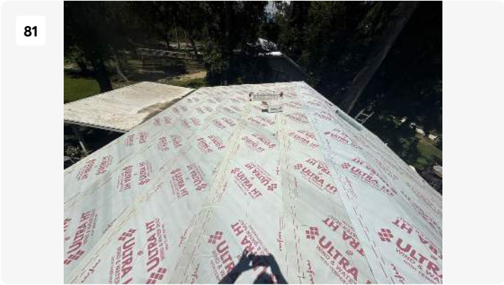
Project: Bruce & Natlie Park - SF GC Work Date: Sep 4, 2025, 1:35 PM Creator: kaleb carson
