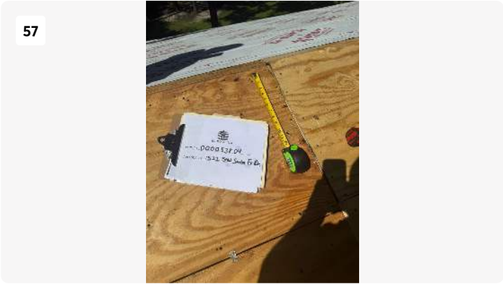
Project: Bruce & Natlie Park - SF GC Work Date: Sep 4, 2025, 11:24 AM Creator: kaleb carson
