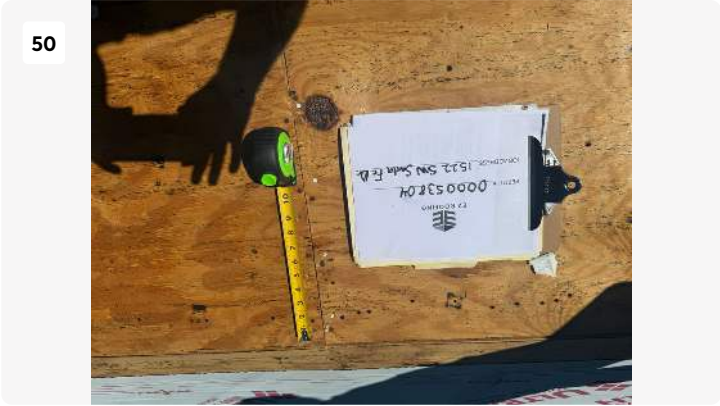
Project: Bruce & Natlie Park - SF GC Work Date: Sep 4, 2025, 11:22 AM Creator: kaleb carson
