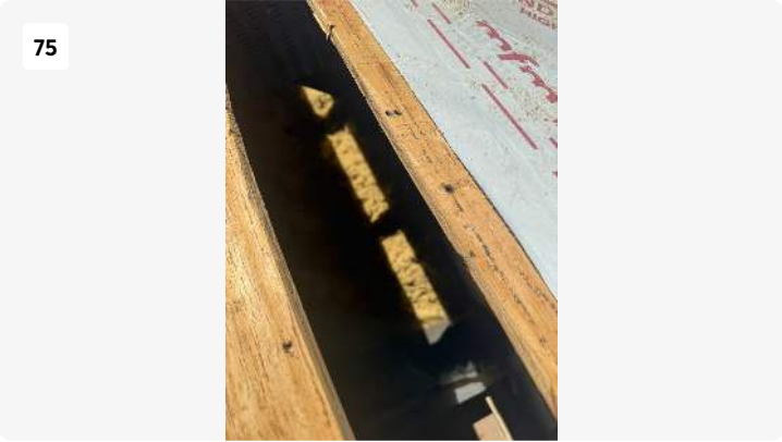
Project: Bruce & Natlie Park - SF GC Work Date: Sep 4, 2025, 12:19 PM Creator: kaleb carson
