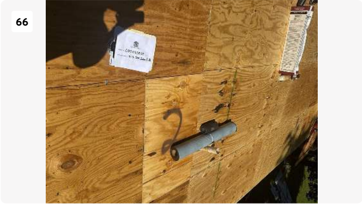
Project: Bruce & Natlie Park - SF GC Work Date: Sep 4, 2025, 11:30 AM Creator: kaleb carson
