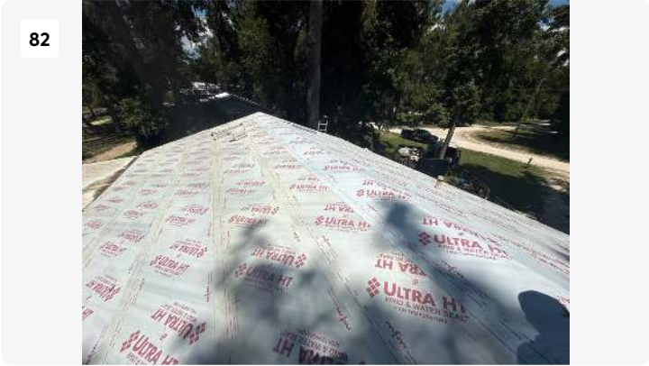
Project: Bruce & Natlie Park - SF GC Work Date: Sep 4, 2025, 1:36 PM Creator: kaleb carson
