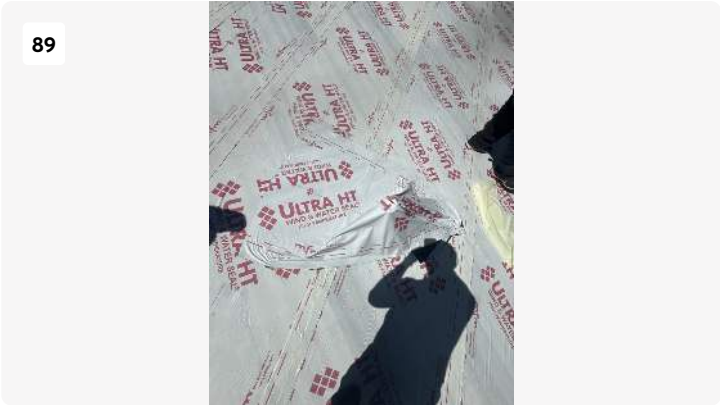
Project: Bruce & Natlie Park - SF GC Work Date: Sep 4, 2025, 1:41 PM Creator: kaleb carson
