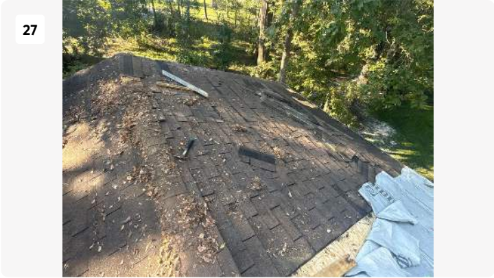
Project: Bruce & Natlie Park - SF GC Work Date: Sep 4, 2025, 9:11 AM Creator: kaleb carson
