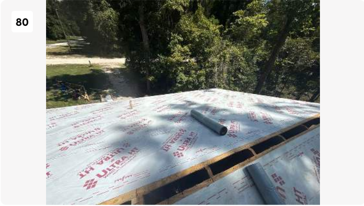
Project: Bruce & Natlie Park - SF GC Work Date: Sep 4, 2025, 1:33 PM Creator: kaleb carson
