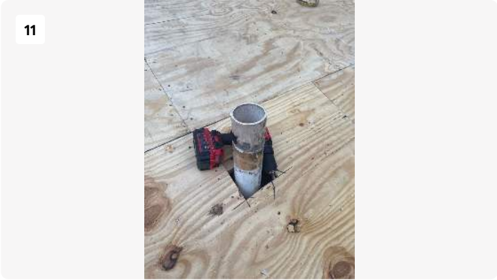
Project: Bruce & Natlie Park - SF GC Work Date: Sep 4, 2025, 8:34 AM Creator: kaleb carson
