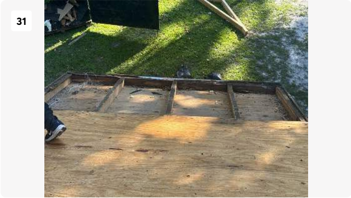
Project: Bruce & Natlie Park - SF GC Work Date: Sep 4, 2025, 9:14 AM Creator: kaleb carson
