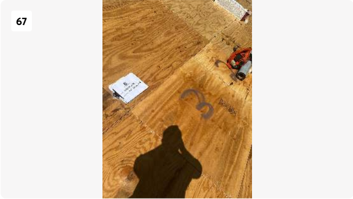
Project: Bruce & Natlie Park - SF GC Work Date: Sep 4, 2025, 12:00 PM Creator: kaleb carson
