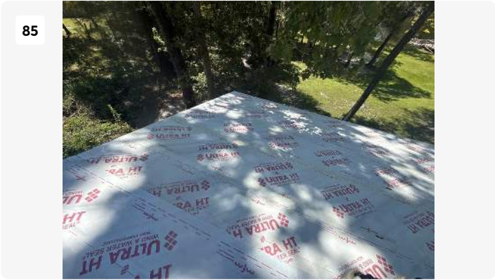
Project: Bruce & Natlie Park - SF GC Work Date: Sep 4, 2025, 1:39 PM Creator: kaleb carson
