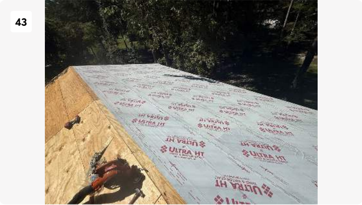
Project: Bruce & Natlie Park - SF GC Work Date: Sep 4, 2025, 11:15 AM Creator: kaleb carson
