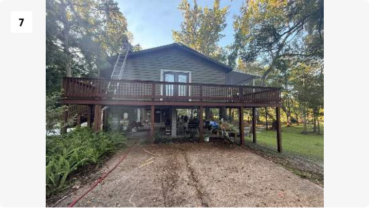
Project: Bruce & Natlie Park - SF GC Work Date: Sep 4, 2025, 8:21 AM Creator: kaleb carson
