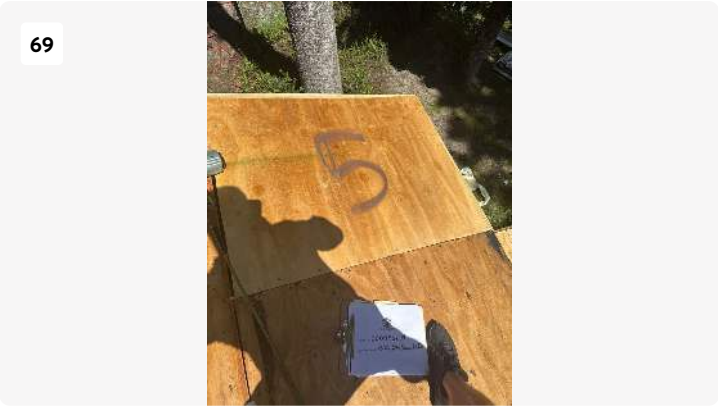
Project: Bruce & Natlie Park - SF GC Work Date: Sep 4, 2025, 12:04 PM Creator: kaleb carson
