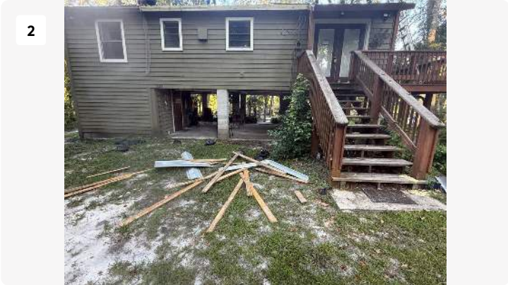
Project: Bruce & Natlie Park - SF GC Work Date: Sep 4, 2025, 8:20 AM Creator: kaleb carson
