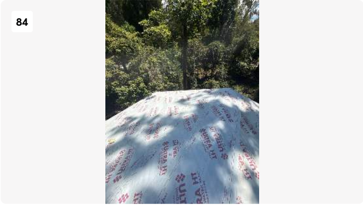
Project: Bruce & Natlie Park - SF GC Work Date: Sep 4, 2025, 1:38 PM Creator: kaleb carson
