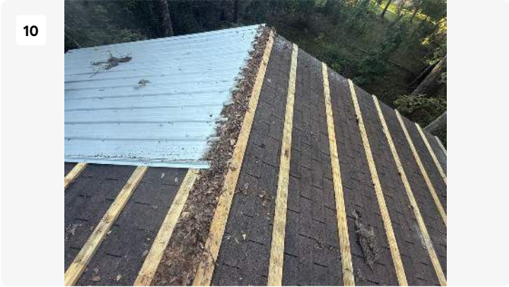
Project: Bruce & Natlie Park - SF GC Work Date: Sep 4, 2025, 8:22 AM Creator: kaleb carson
