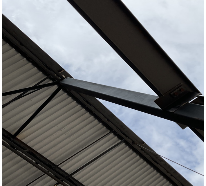
Slip connection at 23/K5 not completed
