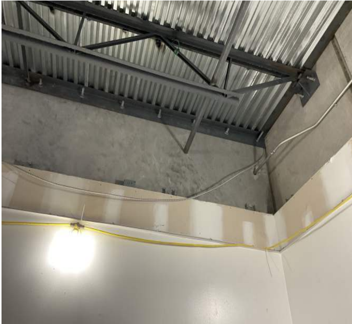
Bridging not anchored in Breakroom Area
