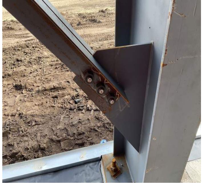
TC bolts at braced frames completed
