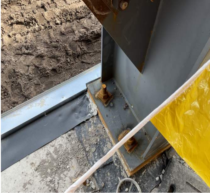
Previously missing plate washer welds completed
