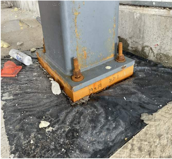
Loose anchor bolts along Line A.8
