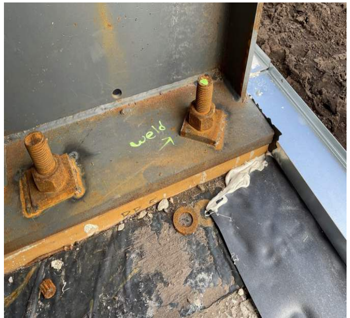
23/E.2 weld missing at plate washer
