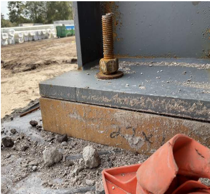
Loose anchors found in several locations along Line 23
