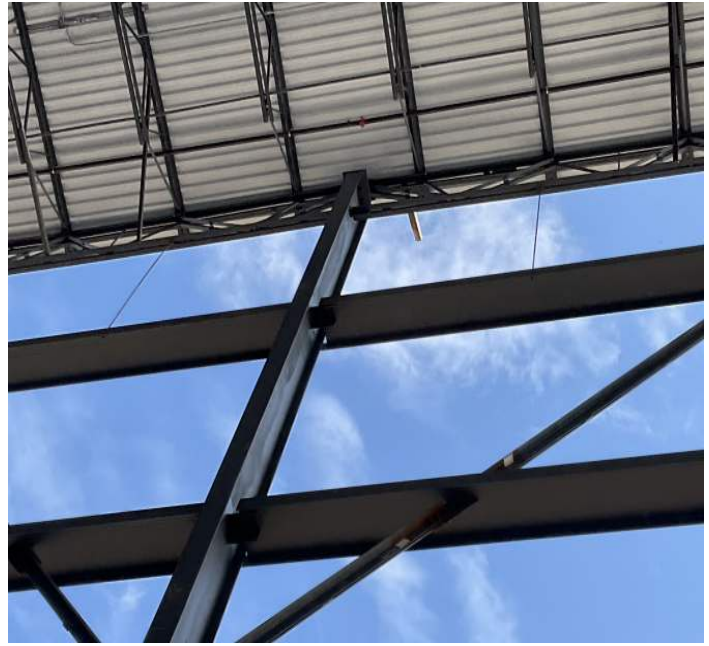
Bottom chords of joists not welded to stabilizer plates per Detail 8/301D
