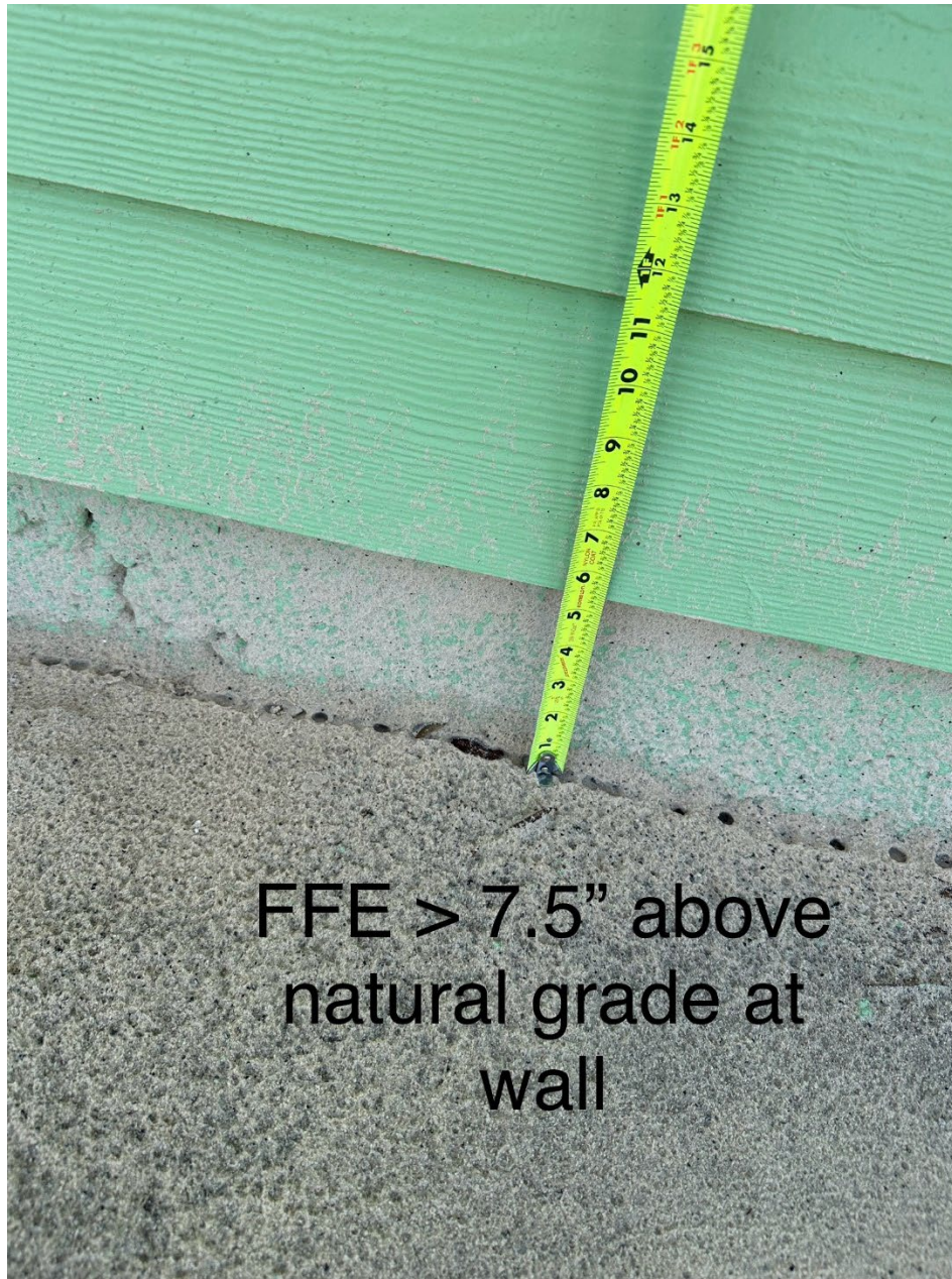
Figure 3. Finished Floor Elevation Greater Than 7.5" Above Finished Grade
