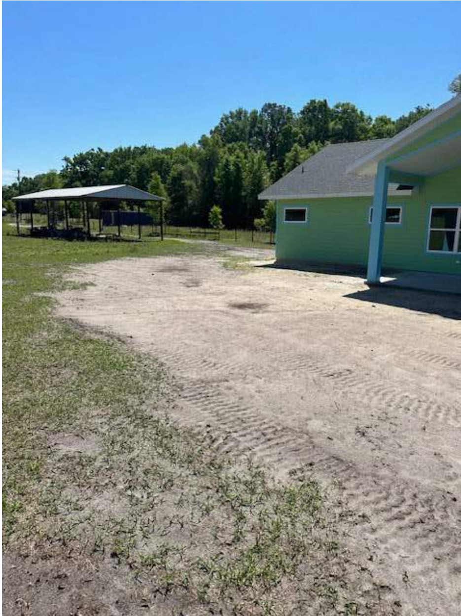
Figure 2. Northeast corner of residence-Swale directs runoff easterly around the residence
