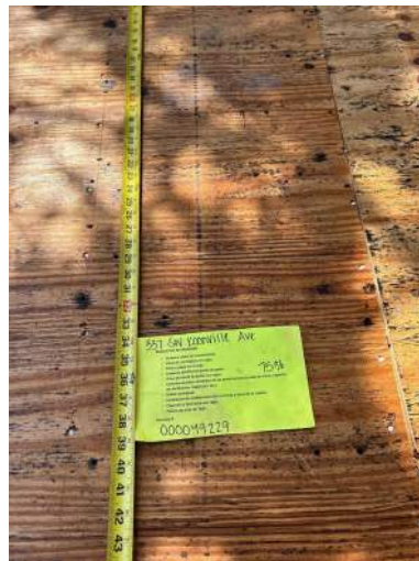
Bannister 7542 Flat Roof 337 SW Koonville Ave • Lake City, FL 32024 Tue, Feb 27 12:29 pm by Jody Simmons
