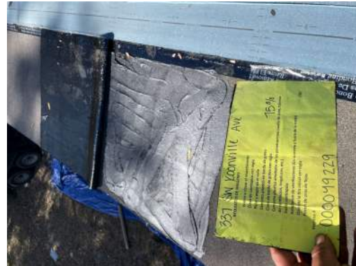
Bannister 7542 Flat Roof 337 SW Koonville Ave • Lake City, FL 32024 Tue, Feb 27 03:44 pm by Jody Simmons
