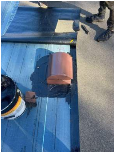
Bannister 7542 Flat Roof 337 SW Koonville Ave • Lake City, FL 32024 Tue, Feb 27 04:27 pm by Jody Simmons
