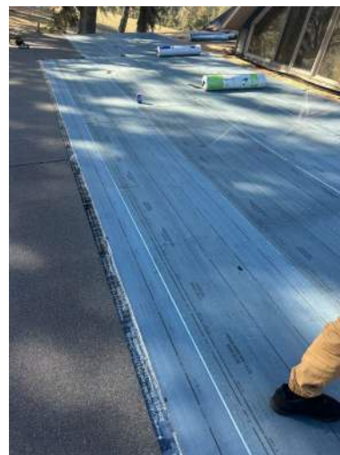
Bannister 7542 Flat Roof 337 SW Koonville Ave • Lake City, FL 32024 Tue, Feb 27 04:26 pm by Jody Simmons
