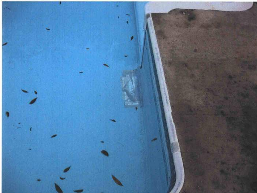
Photograph 2 – View of temporary repair to pool liner
