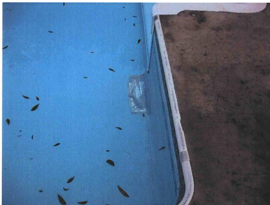
Photograph 2 – View of temporary repair to pool liner
