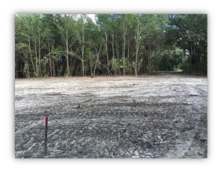
The elevation of the road adjacent to the cleared driveway is 137.00 + 1. The highest existing ground elevation at the foundation is 4.5 below the existing road or 132.50 + 1. The minimum
