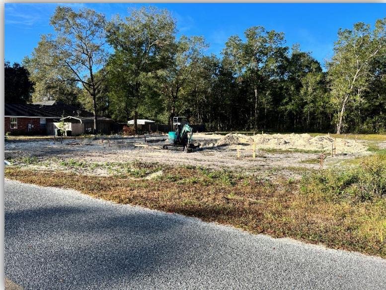
The minimum finished floor elevation shown on the plat is 101.9'. Columbia County LIDAR shows the street centerline elevation to be vary from 98.8' +/- and 99.0' +/- . The minimum
