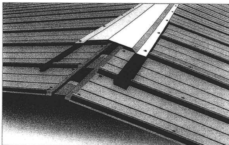
Figure 9 Ridge cap showing outside closure (left) and profile vent (right).
