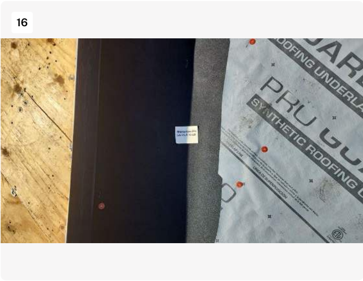
Project: Roofing XL (Ryan) Date: 1/12/2023, 3:51pm Creator: Ryan Boatright
