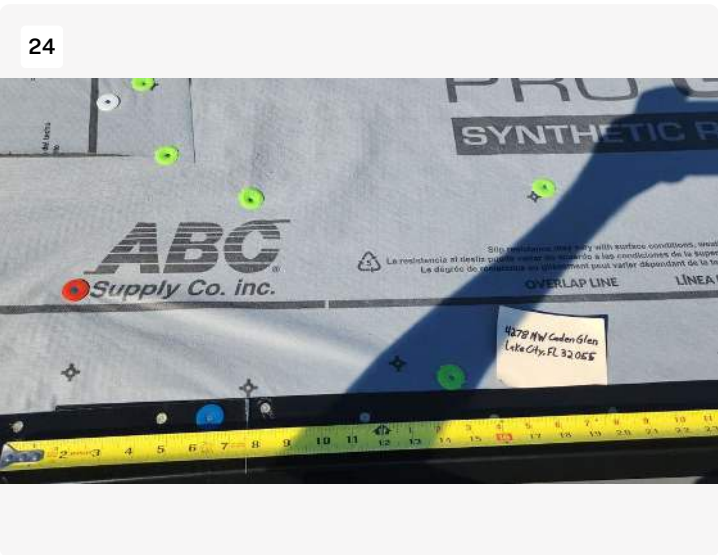
Project: Roofing XL (Ryan) Date: 1/12/2023, 3:56pm Creator: Ryan Boatright
