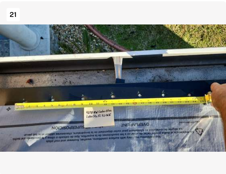
Project: Roofing XL (Ryan) Date: 1/12/2023, 3:55pm Creator: Ryan Boatright
