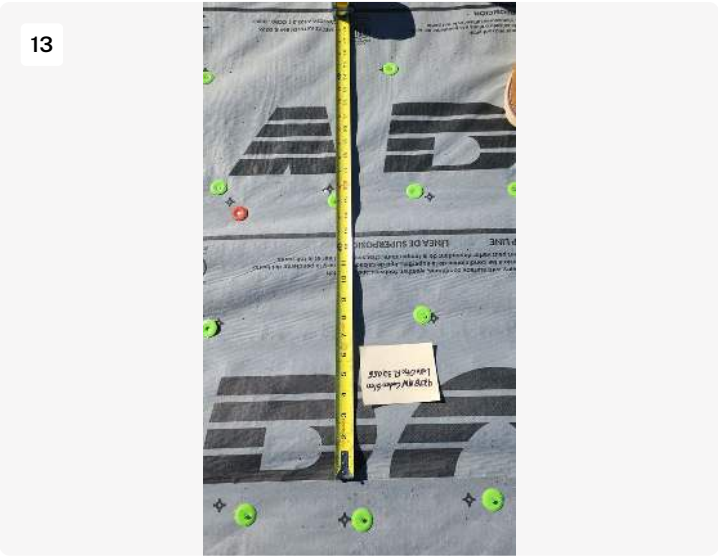
Project: Roofing XL (Ryan) Date: 1/12/2023, 3:50pm Creator: Ryan Boatright
