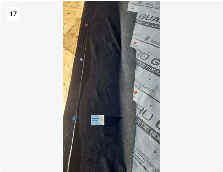
Project: Roofing XL (Ryan) Date: 1/12/2023, 3:52pm Creator: Ryan Boatright
