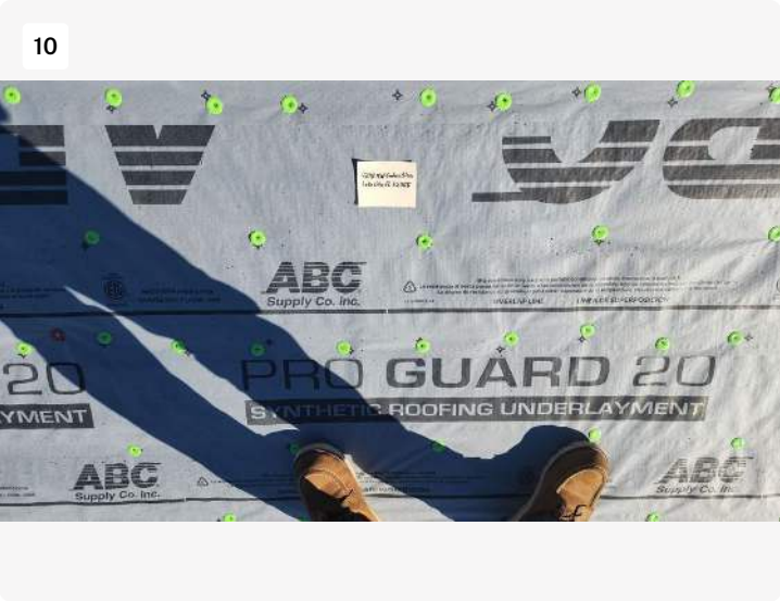
Project: Roofing XL (Ryan) Date: 1/12/2023, 3:49pm Creator: Ryan Boatright
