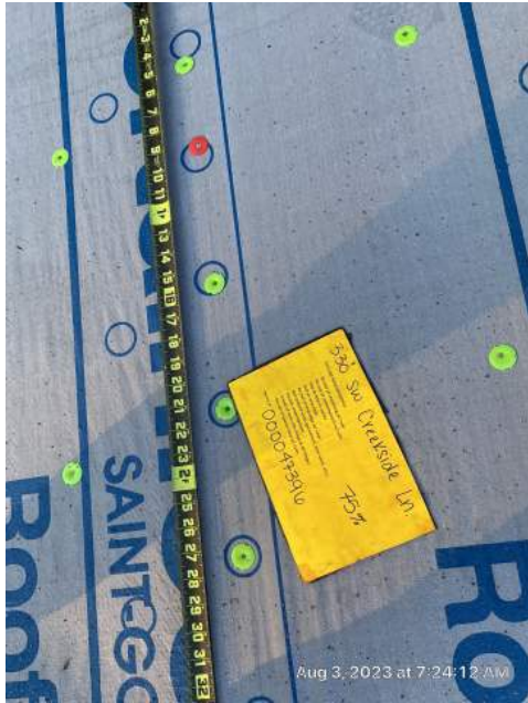
Carruthers 4781 330 SW Creekside Ln • Lake City, FL 32025 Thu, Aug 3 07:24 am by Terry Lewis
