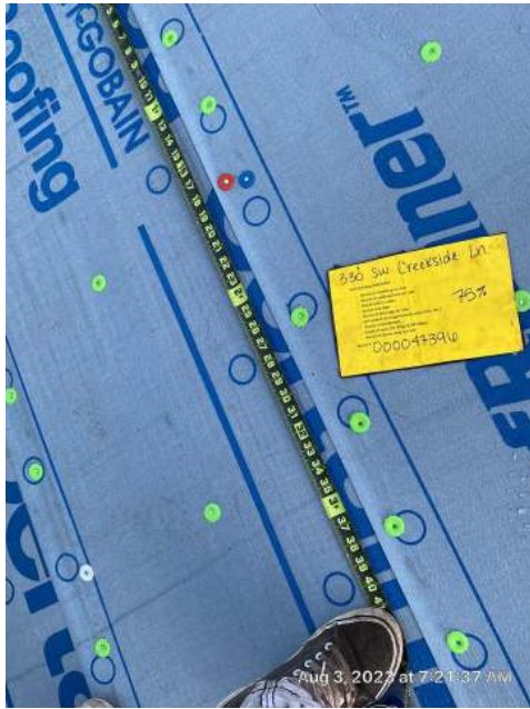
Carruthers 4781 330 SW Creekside Ln • Lake City, FL 32025 Thu, Aug 3 07:21 am by Terry Lewis
