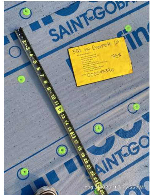
Carruthers 4781 330 SW Creekside Ln • Lake City, FL 32025 Thu, Aug 3 07:23 am by Terry Lewis
