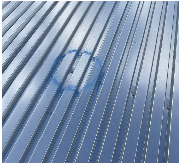
Missing pins and side lap fasteners completed at the roof level
