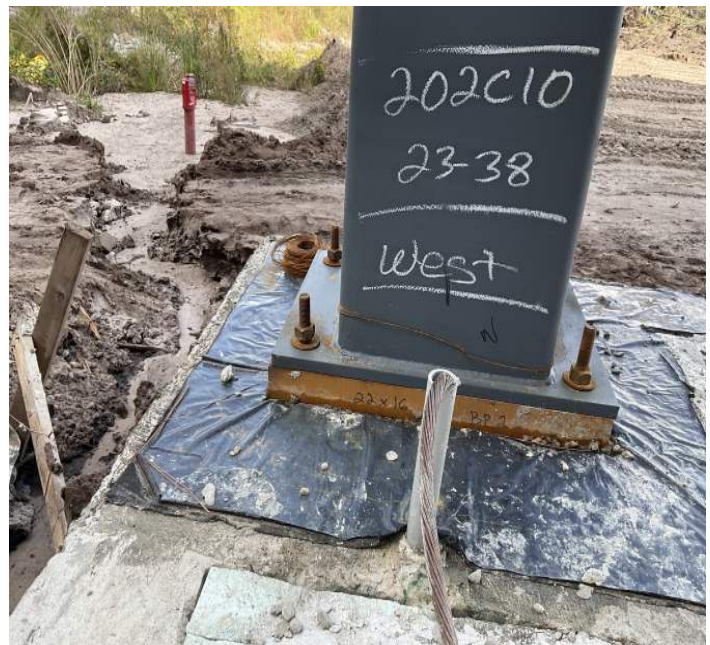
Loose bolts at column base plates
