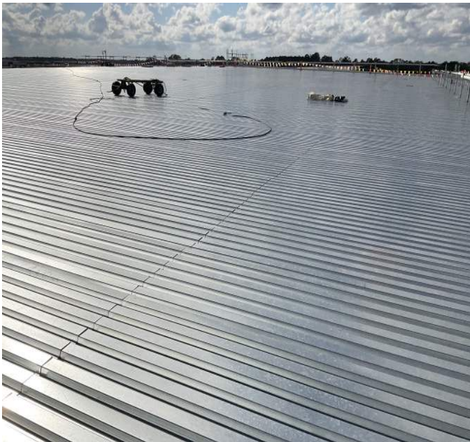
Missing pins and side lap fasteners completed at the roof level
