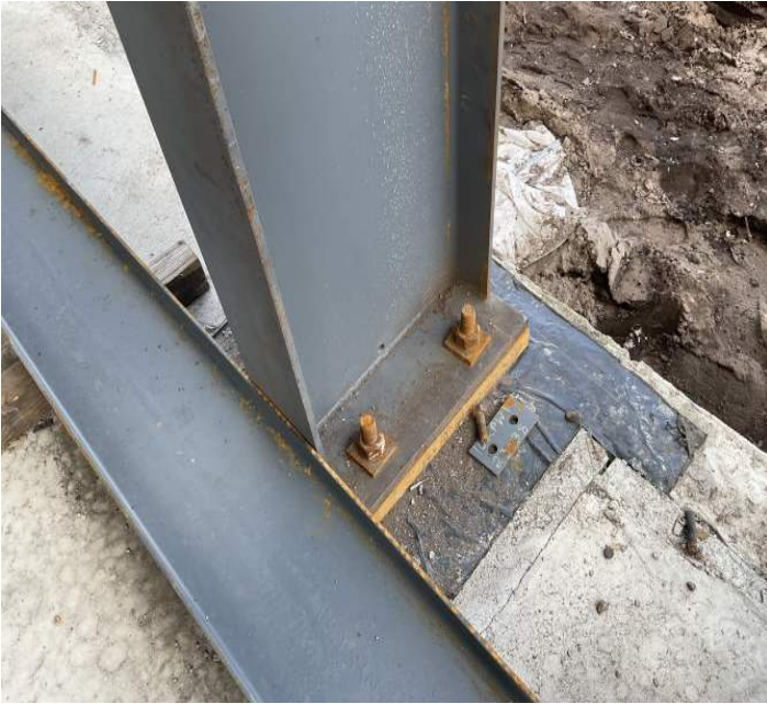
Plate washers not welded along Line 23
