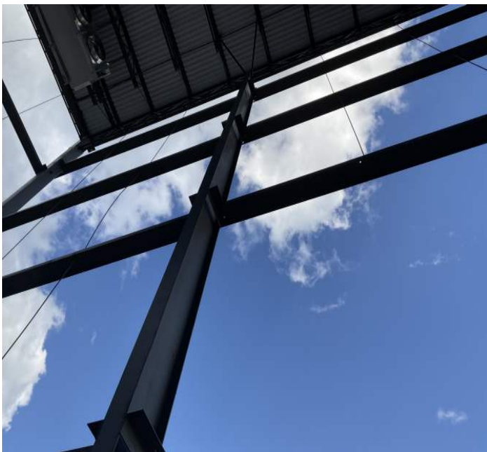
Completed perimeter wind beams along Line 23
