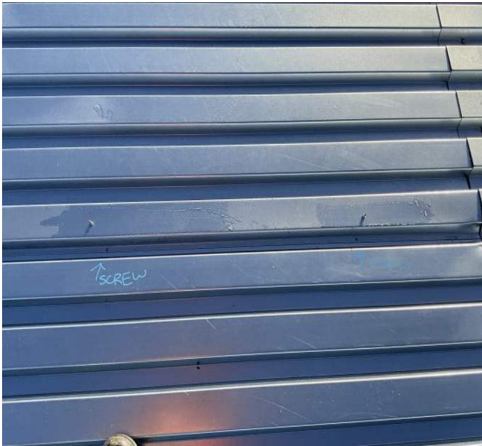
Missing screws completed during inspection
