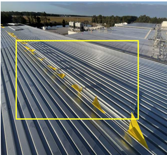
Shot pins missing where decking is stacked on the roof deck
