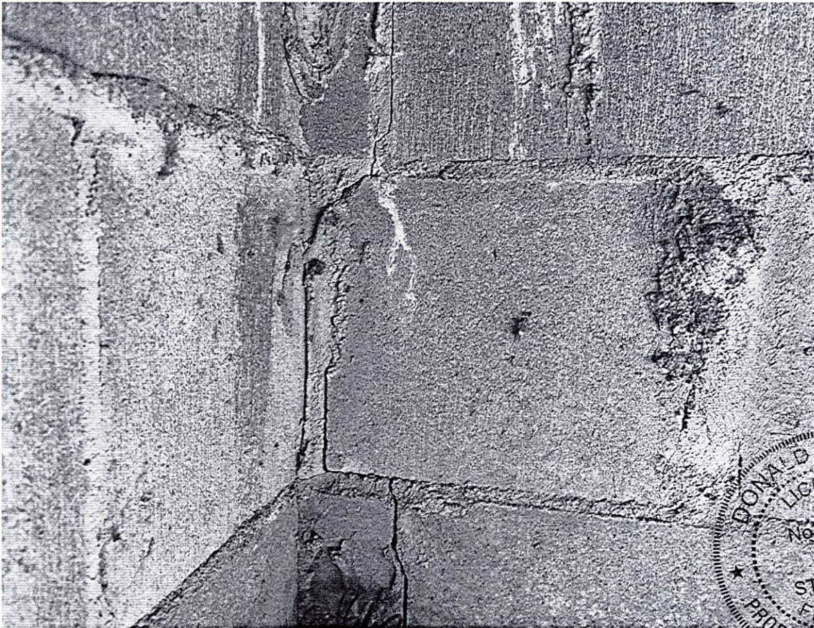
Stairstep cracks in concrete block stem wall as seen in crawl space, due to settlement.
