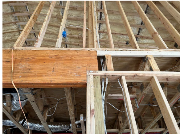
Insufficient Beam Column and Footing (C1)
