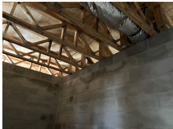
Floor Truss bearing on CMU wall
