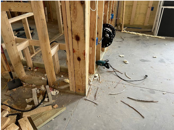
Insufficient Wall Footing (BW1)
