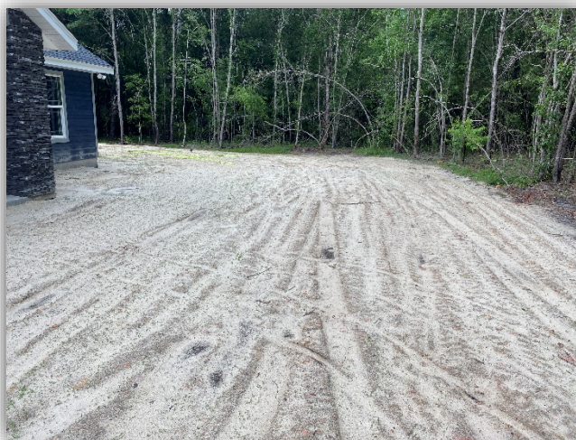
Photo 2. Grading showing positive drainage from the front of the home.
