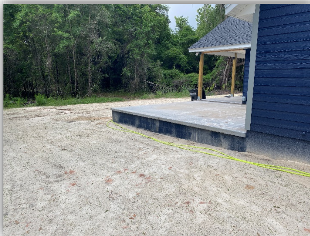
Photo 3. Grading showing positive drainage from the back of the home.
