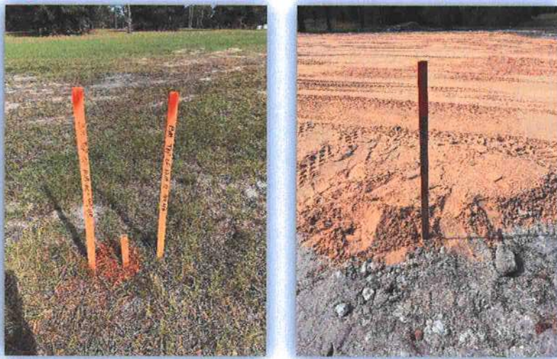
Photo 2. Stake with benchmark & stake at corner of northeast corner of home
