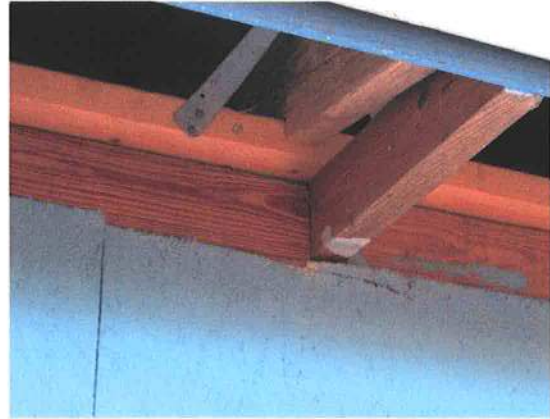
DETAIL AT ADDED BEARING PLATE
