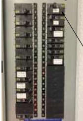
PROPOSED (2) 1P-20A BREAKERS IN POSITION 2 AND 4
