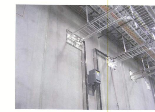
INSTALL TRANSFORMER HIGH ON WALL AND ADJACENT TO VERTICAL WIREWAYS FOR PRIMARY AND SECONDARY CABLE CONNECTS. FLEXIBLE SEALTIGHT CONNECTIONS SHALL BE LESS THAN 3 FEET IN LENGTH.
