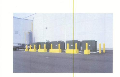
PROVIDE CONCRETE FILLED STEEL BOLLARDS SIMILAR TO THOSE SHOWN IN COORDINATE EXACT LAYOUT AND INSTALLATION REQUIREMENTS WITH AN AUTHORIZED REPRESENTATIVE OF THE LOCAL UTILITY COMPANY.
