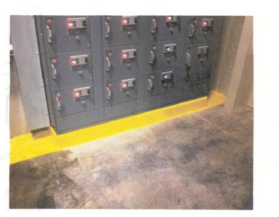
EXAMPLE OF A SATISFACTORY INSTALLATION FOR MOTOR CONTROL CENTER ON RAISED CONCRETE PAD. EXPOSED CONCRETE SHALL NOT BE MORE THAN AS SHOWN IN THIS PHOTO.
