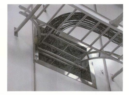
INSTALL CABLES TO SIDES OF TRAY IN A NEAT MANNER ON CABLE TRAY AND TIE DOWN IN SETS AS SHOWN IN THIS PHOTOGRAPH.
