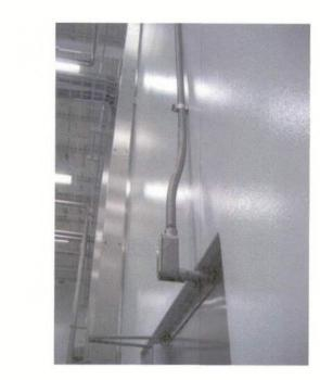
PROVIDE TWO HOLE, STAND OFF STRAPS FOR VERTICAL CONDUITS DROPS TO SECURITY DEVICES AS SHOWN IN THIS PHOTOGRAPH. PROVIDE STAINLESS STEEL CONDUITS, STRAPS AND HARDWARE IN ALL PROCESS AREAS FOR DROPS TO DEVICES. DO NOT PAINT CONDUITS OR BOXES. COORDINATE SECURITY REQUIREMENTS AND PREPARE FRAMES AND DOORS
