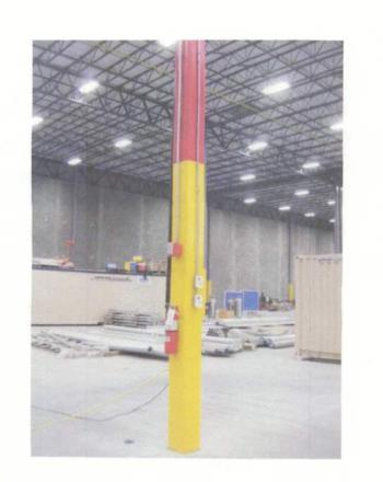
PROVIDE TWO HOLE, STAND OFF STRAPS FOR VERTICAL COMDUITS DROPS ON COLUMNS AS SHOWN IN THIS PHOTOGRAPH. PROVIDE STAINLESS STEEL CONDUITS, STRAPS AND HARDWARE IN ALL PROCESS AREAS FOR DROPS TO DEVICES. DO NOT PAINT CONDUITS OR BOXES.
