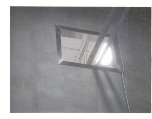
DO NOT INSTALL VERTICAL CONDUITS WITH OFFSETS AS SHOWN IN THIS
