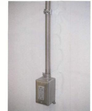
PROVIDE FS BOXES IN ALL AREAS. INSTALL VERTICAL CONDUITS WITHOUT OFFSETS AS SHOWN IN THIS PHOTOGRAPH. PROVIDE STAINLESS STEEL CONDUITS AND BOXES IN ALL PROCESS AREAS FOR DROPS TO DEVICES.
