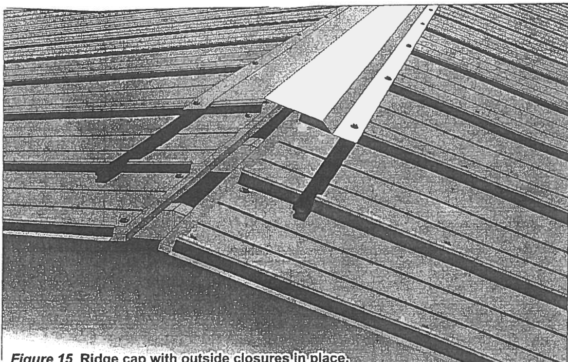
Figure 15 Ridge cap with outside closures in place.
