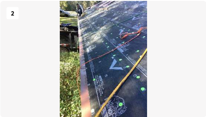
Project: Michael McKee #8170 Truss Repairs. Engineering in the file.. $1550 for engineering. Date: 1/24/2025, 11:45am Creator: Thomas Grigsby
