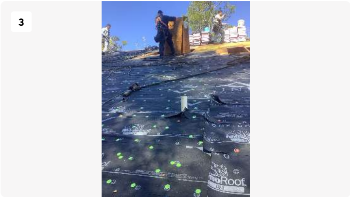
Project: Michael McKee #8170 Truss Repairs. Engineering in the file.. $1550 for engineering. Date: 1/24/2025, 11:46am Creator: Thomas Grigsby
