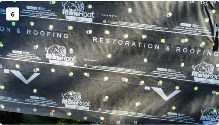
Project: Michael McKee #8170 Truss Repairs. Engineering in the file.. $1550 for engineering. Date: 1/24/2025, 11:34am Creator: Thomas Grigsby
