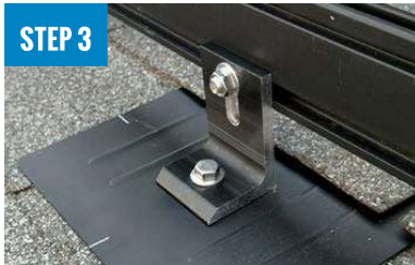
STEP 3 ATTACH L-FOOT TO RAIL
