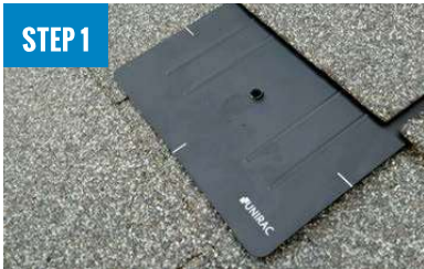
STEP 1 INSTALL FLASHKIT PRO FLASHING
