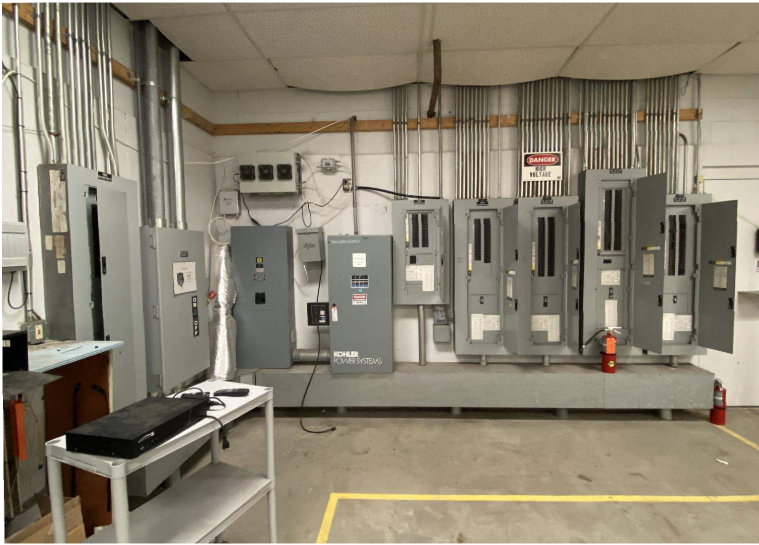
① EXISTING ELECTRICAL TO BE DEMOLISHED
