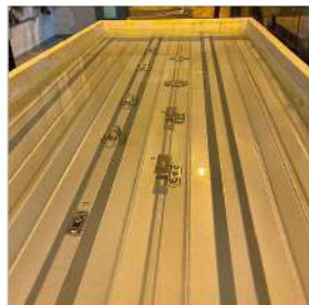
Photo No. 1 System 01
